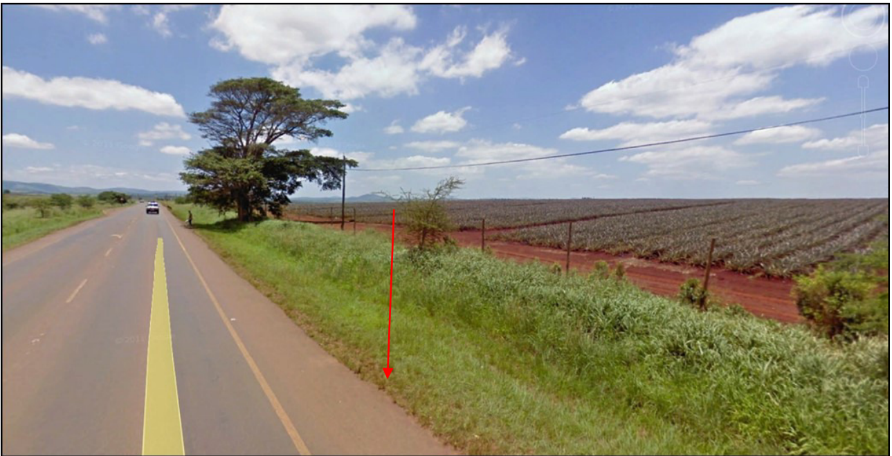
Plate 5-4: The approximate tie-in point of the intersection road from the realigned R22, to the existing R22 (Ref: Google Earth 2016).
