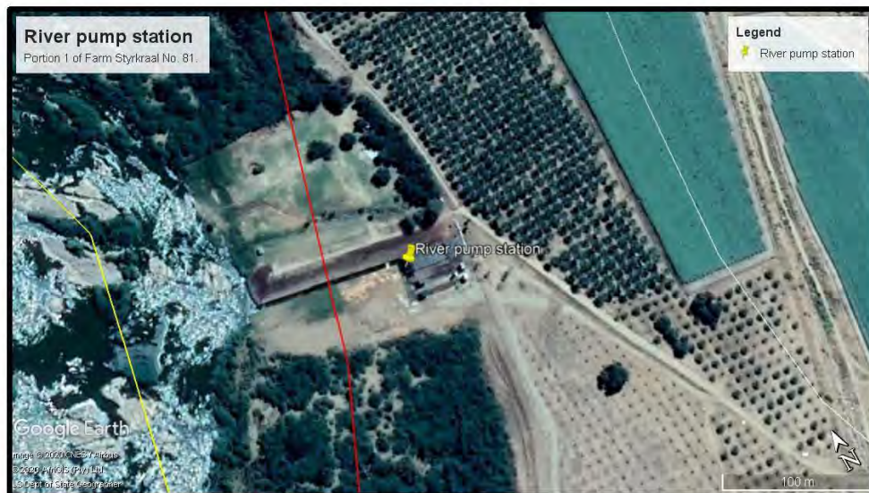
Figure 5: River pump station
