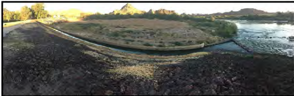
Figure 7: River intake structure
