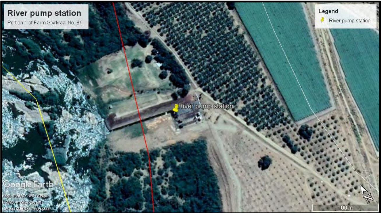
Figure 7: River pump station
