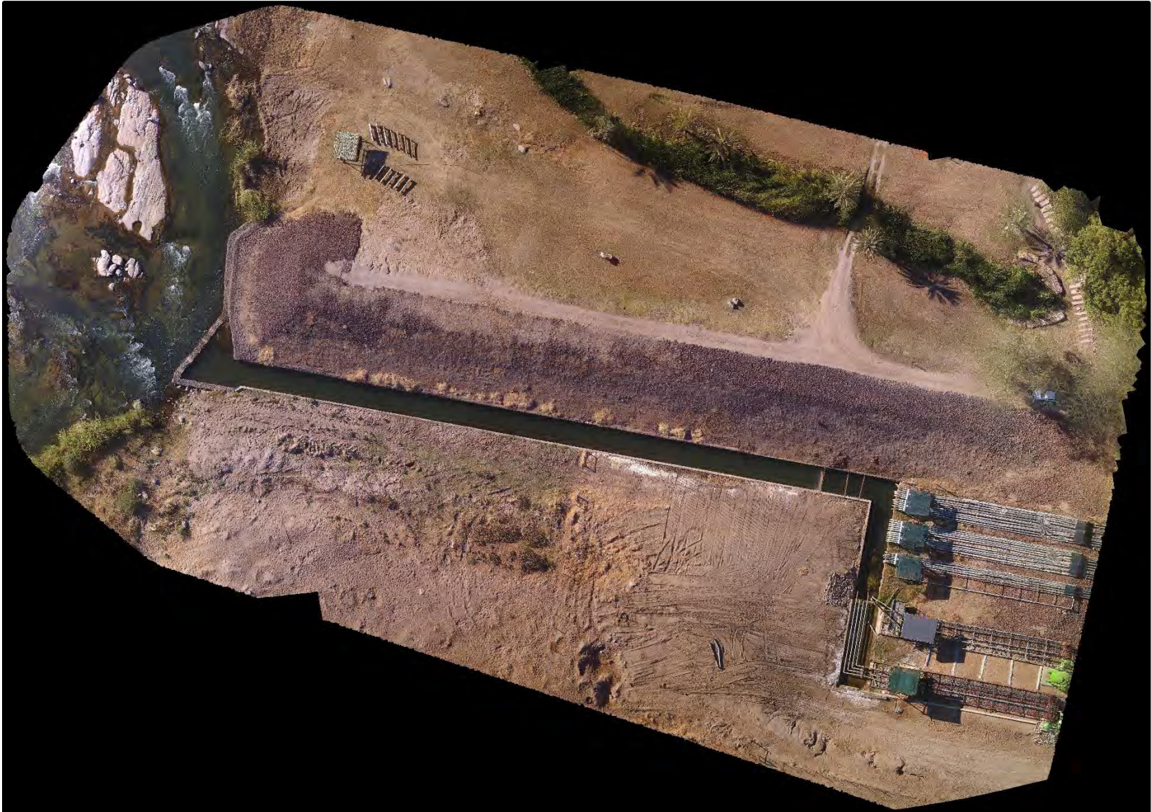
Drone footage of the intake structure
