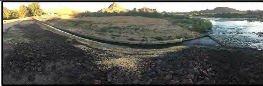
Figure 6: River intake structure
