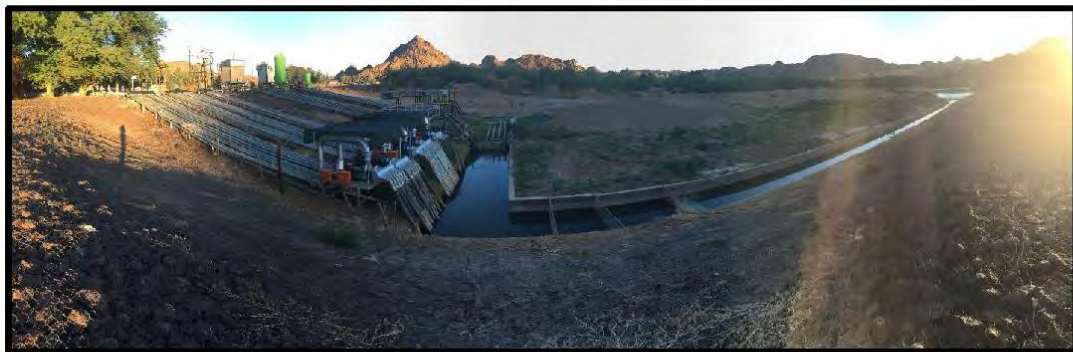
Figure 5: Intake and river pump station
