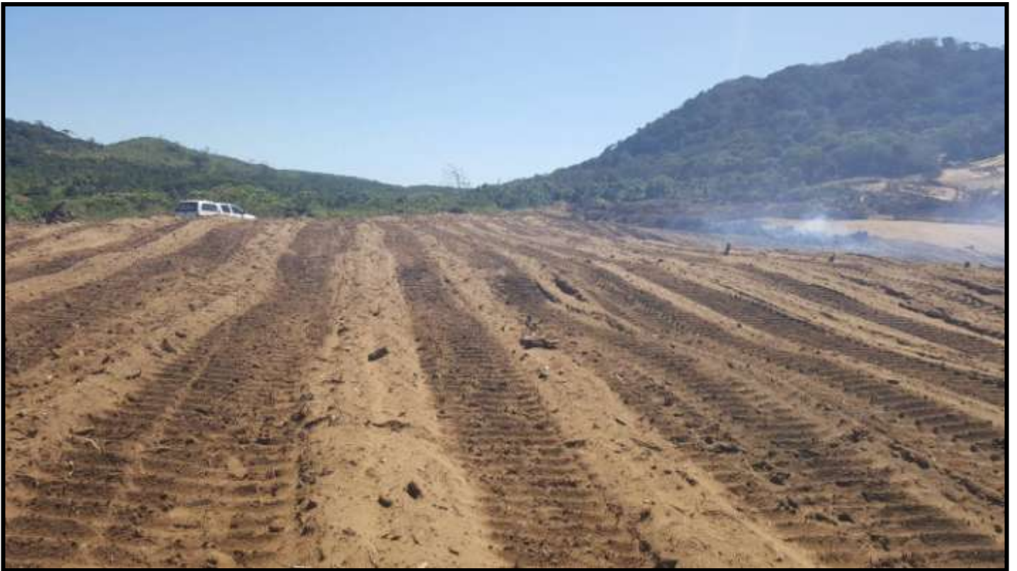
Fig. 17: Cleared Area At RD036
