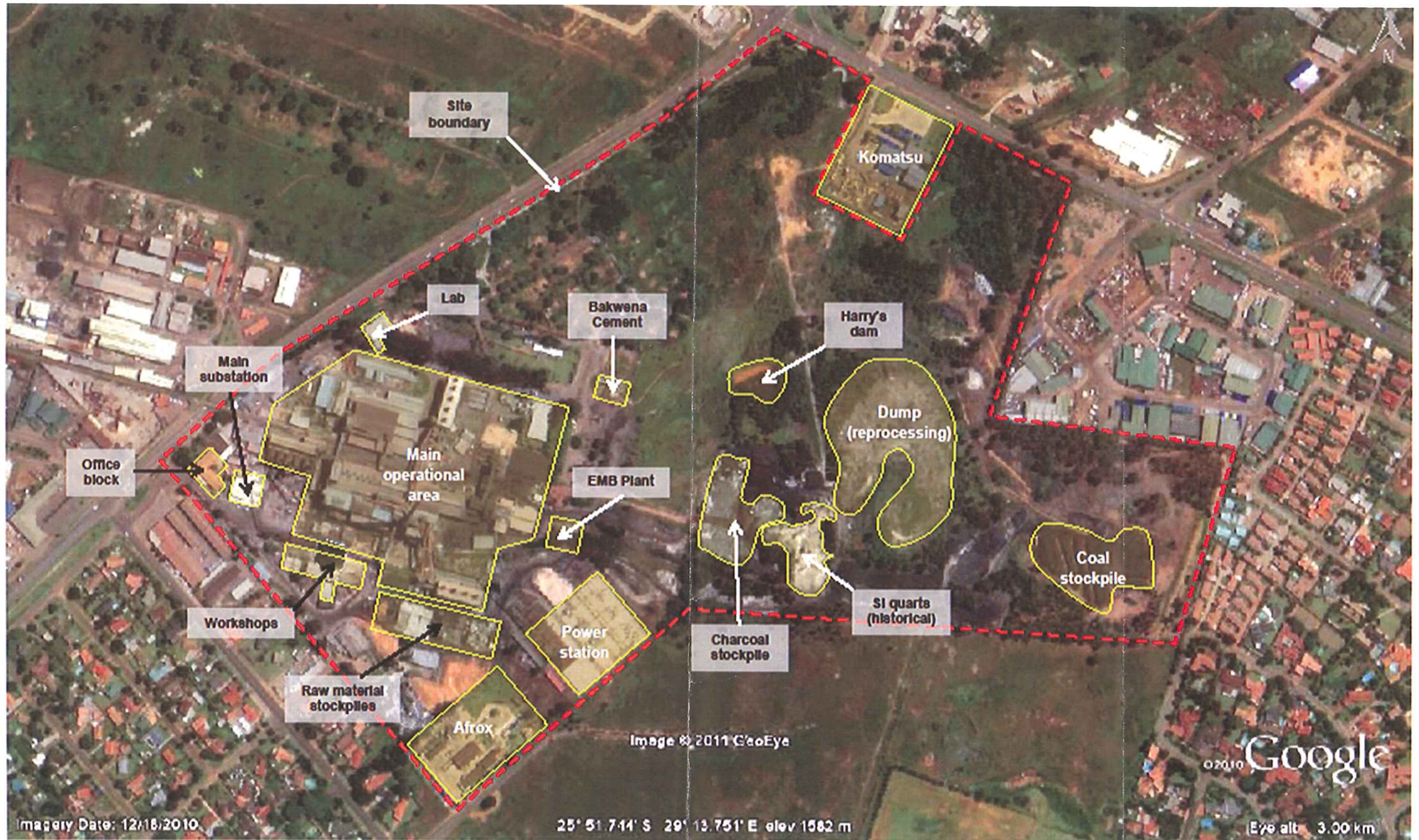
Figure 1-3: General site layout using Google Earth™ image
