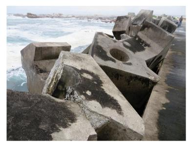
Figure 65: Broken concrete armour units along the southern breakwater
