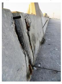
Figure 68: Reinforcement exposed along the western breakwater crest wall
