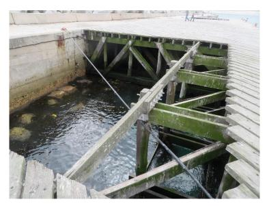
Figure 59: Sub-structure and additional bracing cable of the timber quay
