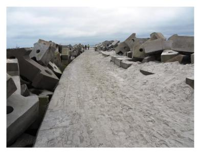
Figure 61: Windblown sand accumulated on the eastern breakwater
