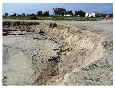
Figure 46: Eroded area behind the rock revetment
