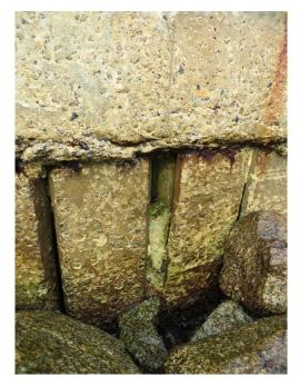
Figure 27: Separation of the concrete sheet pile walls
