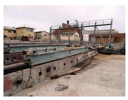
Figure 71: Slipway support beams and cradle
