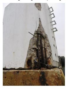
Figure 82: Exposed reinforcement of navigation aid support structure
