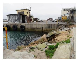
Figure 84: Evidence of the rubble revetment deteriorating
