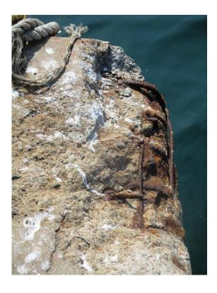
Figure 9: Exposed reinforcement at NE corner of Jetty 2
