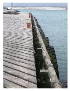
Figure 60: Bollard and tyre fender system on the timber quay
