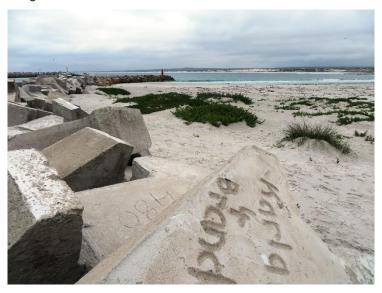
Figure 62: Sand build-up along the armour units of the eastern breakwater
