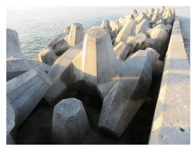
Figure 67: Different type of armour units used along the western breakwater
