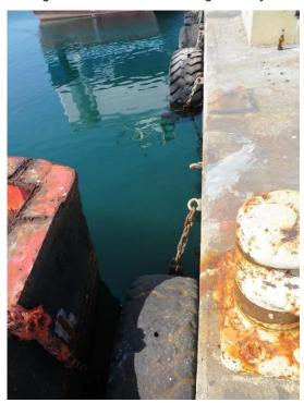
Figure 13: Missing tyre fender at Jetty 4
