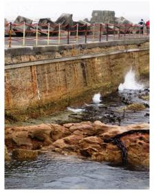
Figure 64: Evidence of water penetrating through the southern breakwater structure
