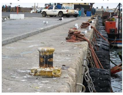
Figure 56: Tyre fenders and bollards along the main quay
