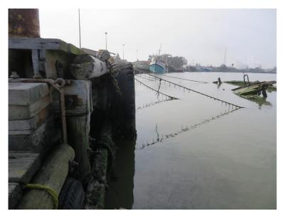
Figure 36: Tyre fender and sunken vessel at the western end of the quay
