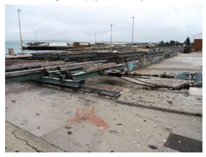
Figure 73: Slipway vessel support beams
