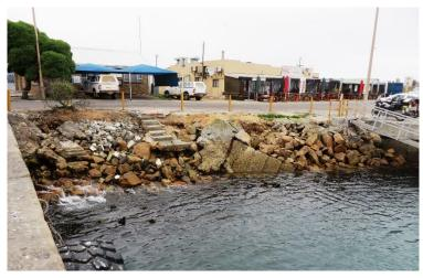
Figure 83: Rubble revetment between main and secondary quays
