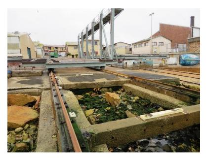
Figure 72: Slipway cradle and rail system
