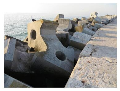
Figure 66: Concrete armour units along the western breakwater
