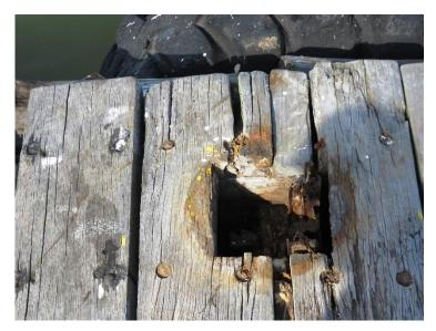
Figure 38: Missing bollard on timber quay
