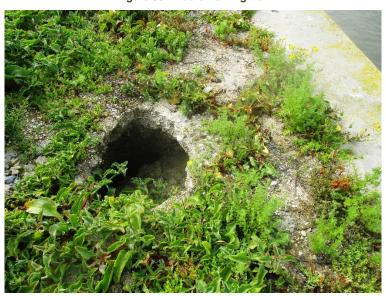
Figure 31: Sink hole alongside middle training wall
