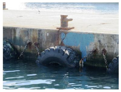
Figure 11: Crack below steel bollard on Jetty 3
