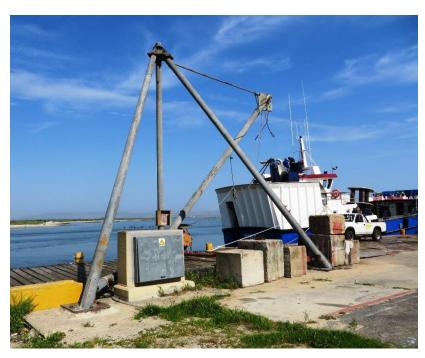
Figure 40: Broken shear-leg crane on eastern end of timber quay
