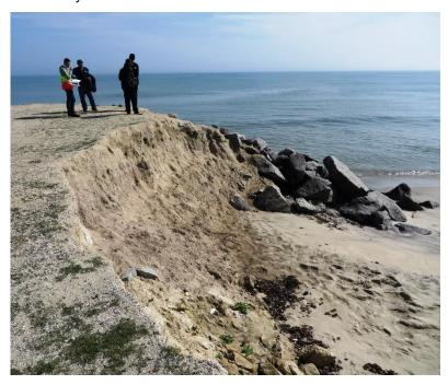
Figure 45: Coastal erosion adjacent to the rock revetment
