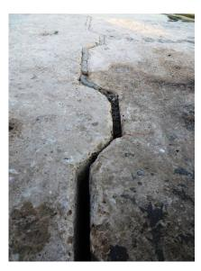
Figure 69: Evidence of previous grouting repairs in the western breakwater joints
