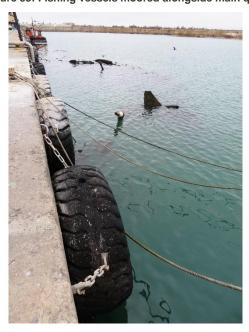
Figure 54: Sunken vessels alongside main quay occupying quay space
