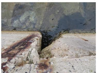
Figure 70: Water penetrating through crack in western breakwater structure (looking down the inner face of the breakwater towards the water)
