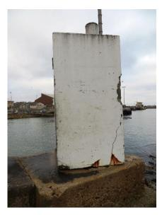
Figure 81: Damaged navigation aid (a.k.a. Lighthouse)
