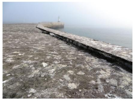
Figure 26: Eastern breakwater and evidence of concrete deck settlement
