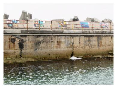
Figure 63: Water penetrating through a crack in the southern breakwater
