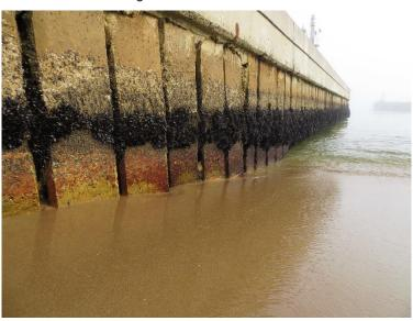
Figure 29: Separated and misaligned sheet pile walls
