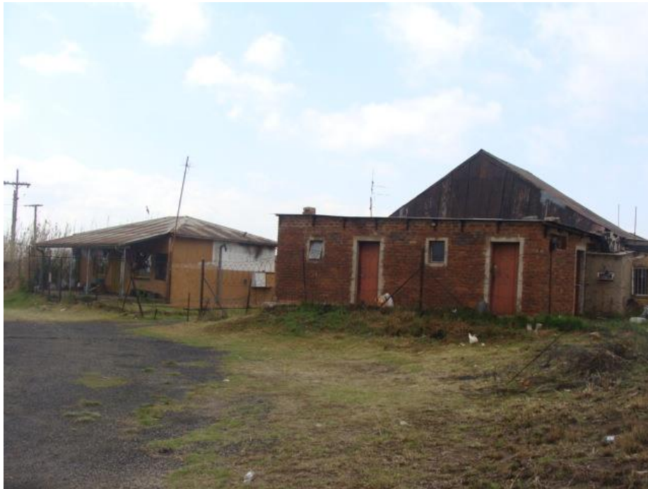
Figure 13 Some of the buildings at site no. 4.
