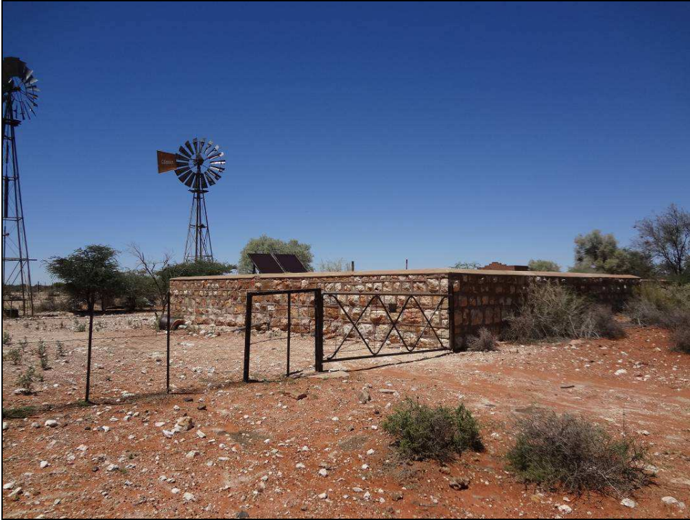
Fig.14 Stone kraal, solar panels & water installation at Point S9, Sanddraai 391.
