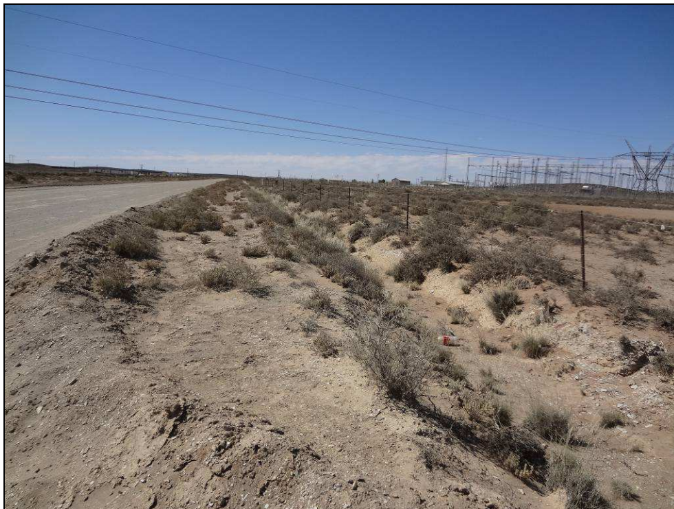
Fig.2 Helios Sub-station as seen from Point C.
