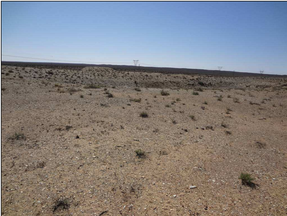
Fig.6 Point B near Eskom Helios Sub-station.
