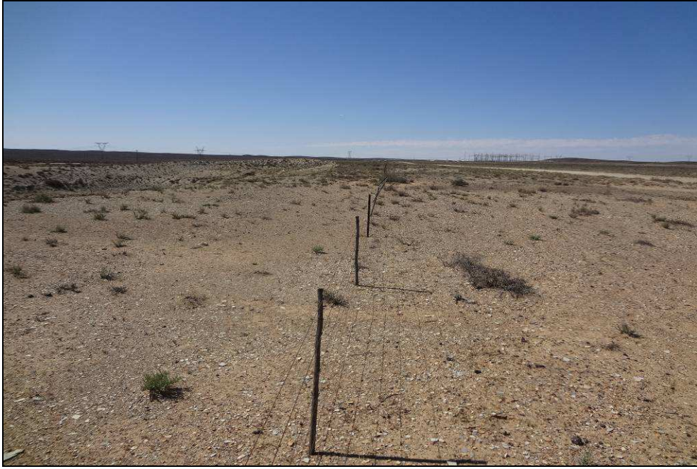
Fig.5 Point B near Eskom Helios Sub-station.
