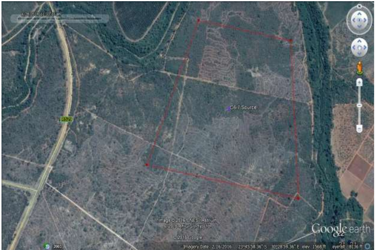
Fig.26: Aerial view of G6/7 location (Google Earth 2016).
