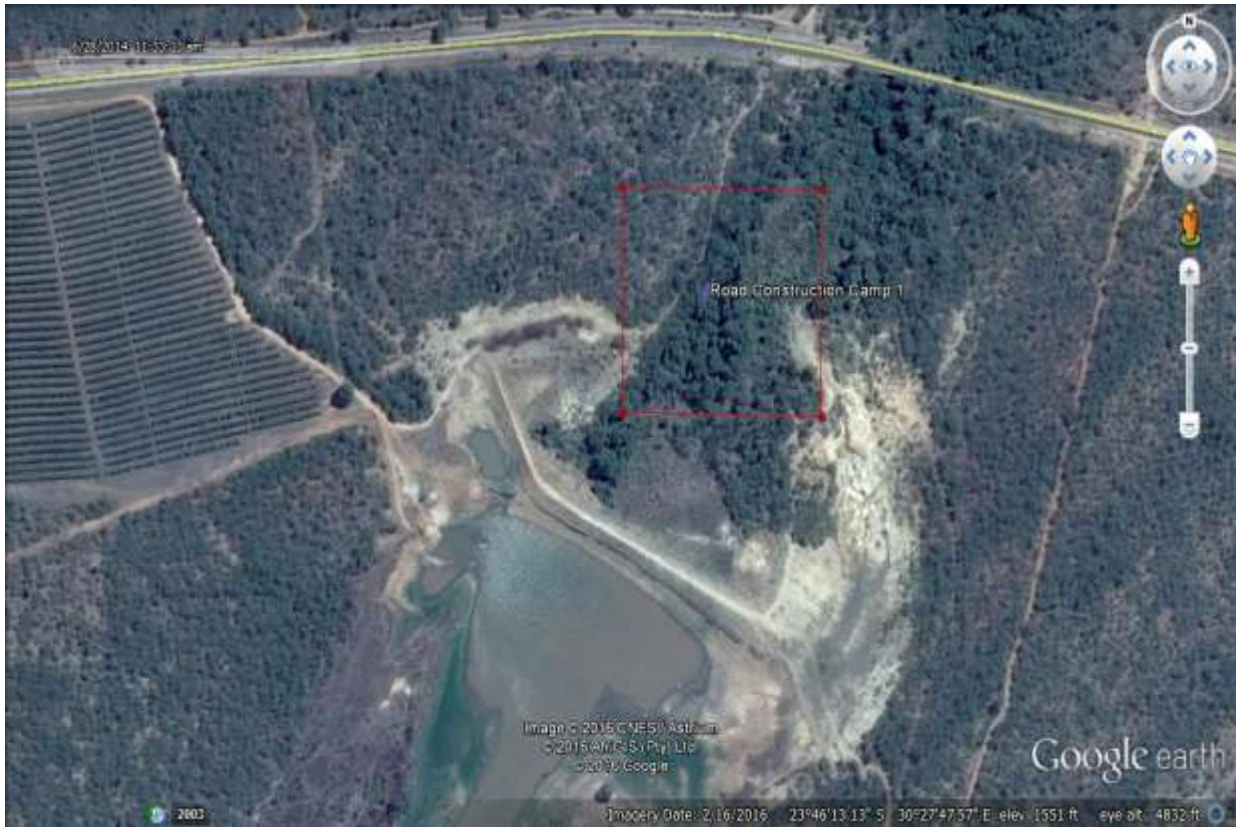
Fig.23: Aerial view of Road Construction Camp 1 location (Google Earth 2016).
