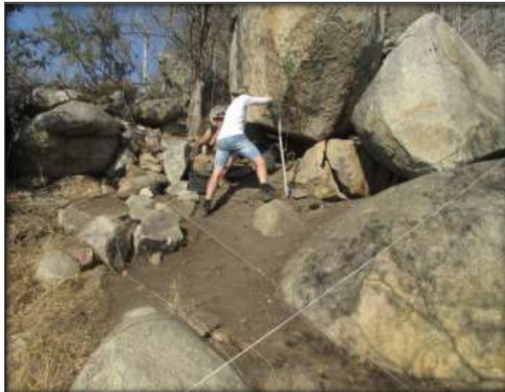
Fig.26: Surface cleaning in progress at Block 1.
