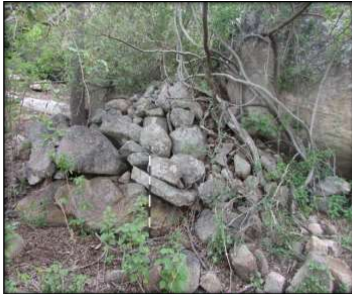
Fig.6: Some of terrace walling at the site.
