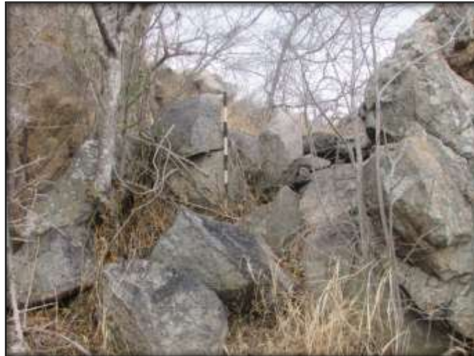
Fig.33: Another section of terrace walling.
