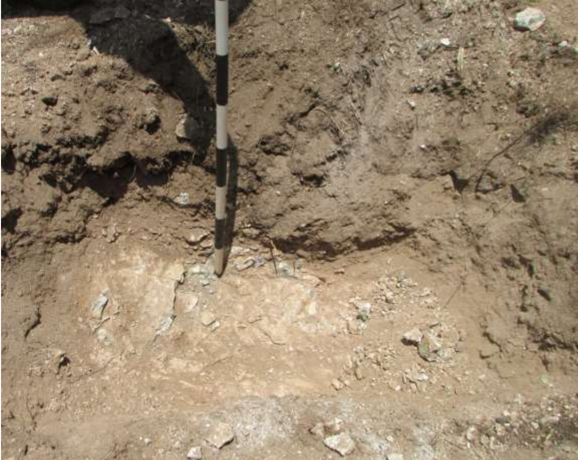
Figure 14: The stratigraphy in the trench consists of loose top soil on top of a layer of undisturbed bed rock (weathered sandstone) at a depth of around 0.50m below the PSL.
