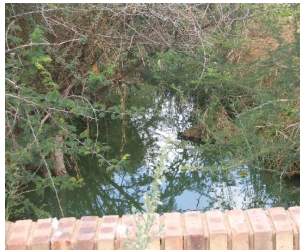
Discharge to the nearest stream
