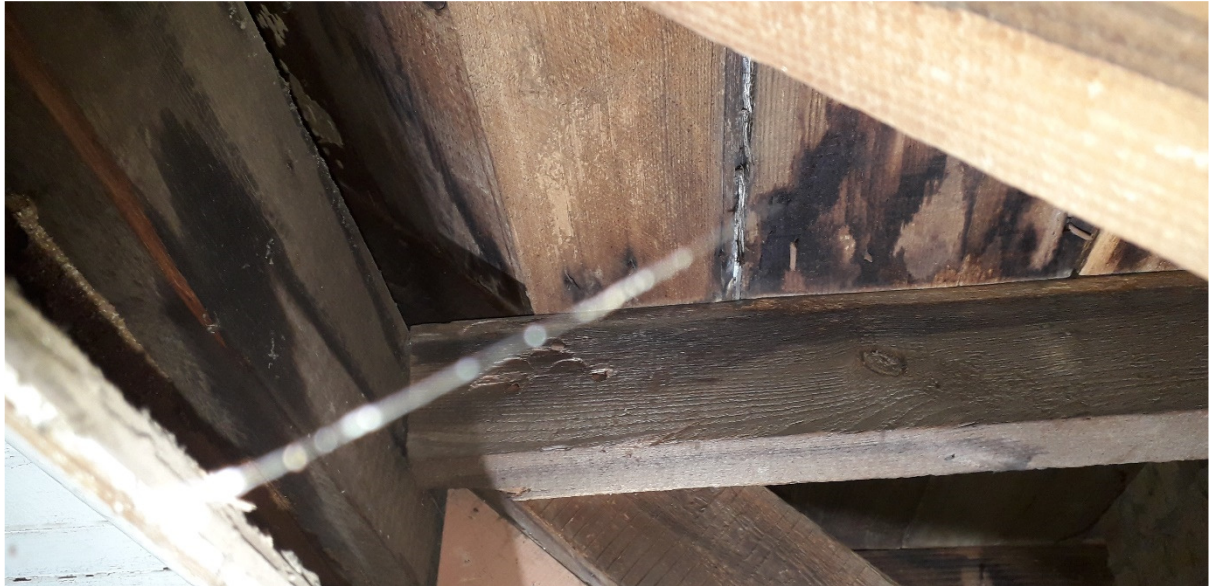
Underside of box gutter above the library
