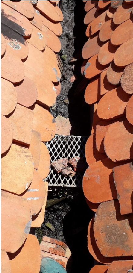
RHS central box gutter and channel above the library
