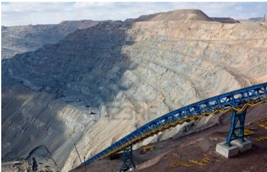
Figure 6: Example of a conveyor utilised for spoil transportation.
