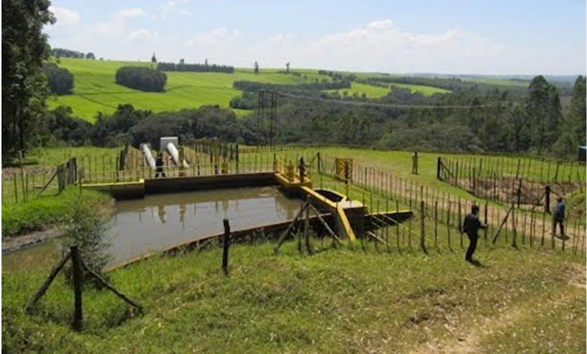
Figure 2: Forebay. (Note for the proposed project this structure will measure as much as 20m x 20m in plan.)
