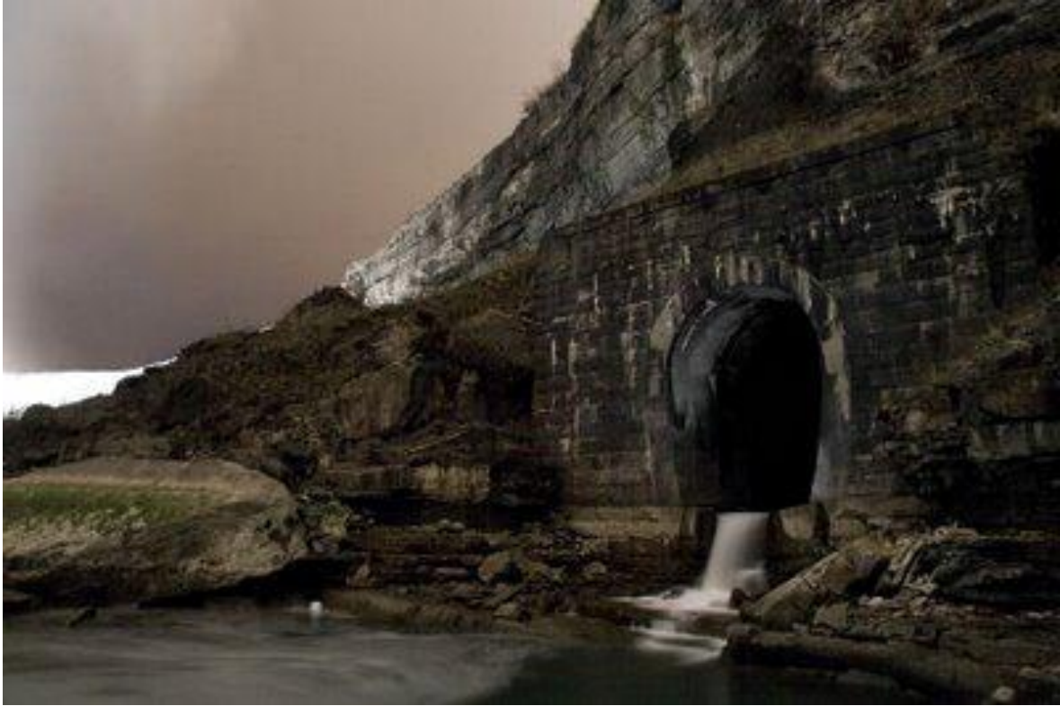
Figure 4: Outfall from the underground power station. (Note for the proposed project this infrastructure would be smaller, approximately 4m in diameter.)
