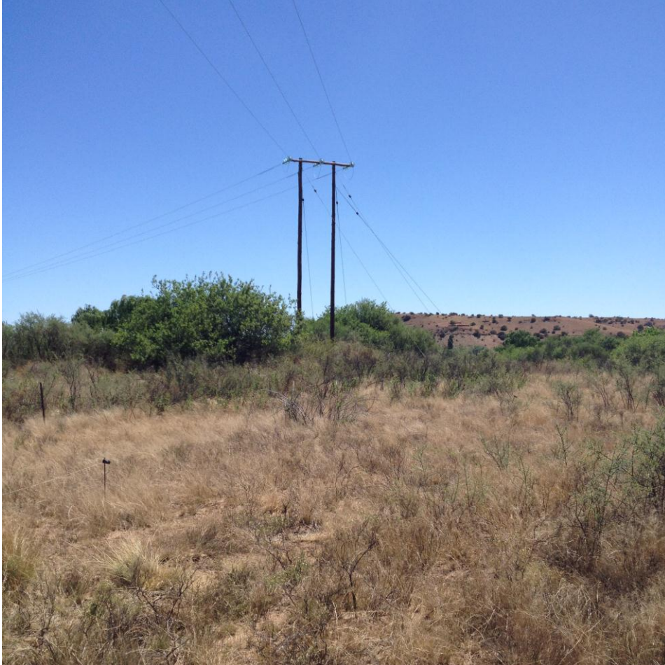
Image 11: Existing power line to be dismantled
