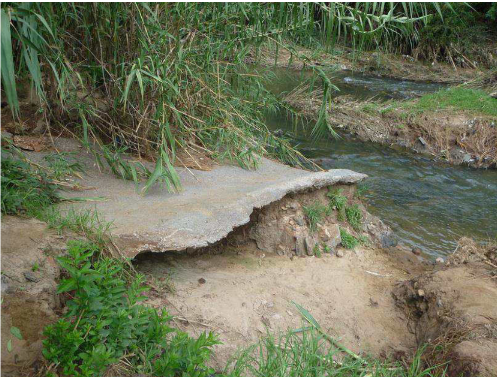
Figure 16 Human impacts (old storm water structures?) and erosion/sedimentation on the eastern banks of the Rietspruit at the end of Poole Avenue
