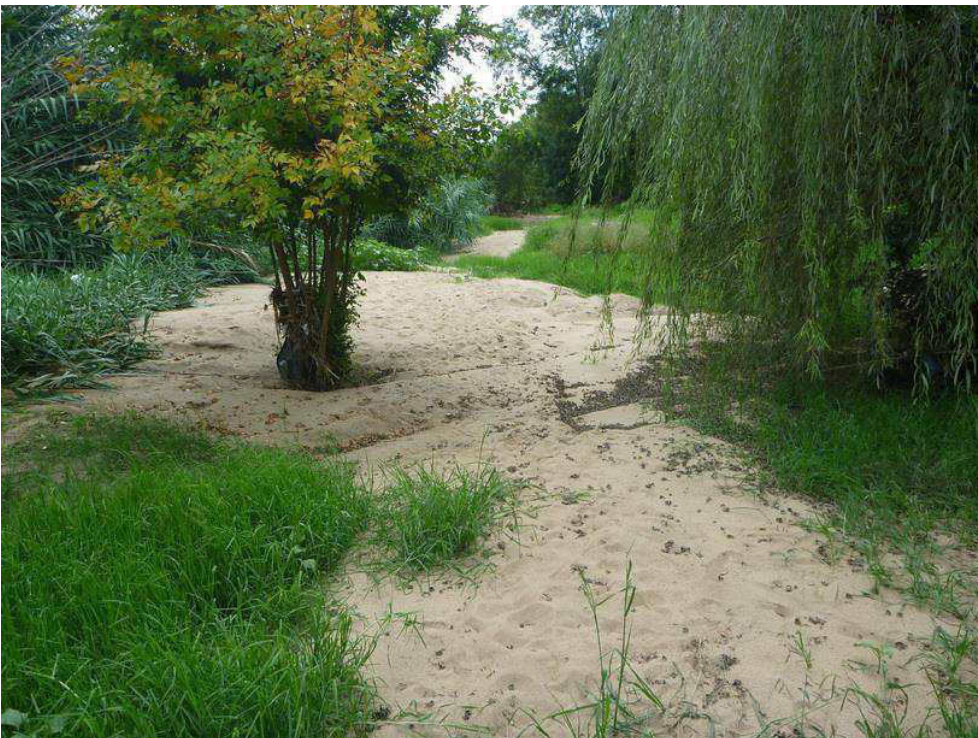
Figure 18 Significant sedimentation (of granitic origin from upstream of the survey site) within the drainage channel the Rietspruit near the end of Poole Avenue
