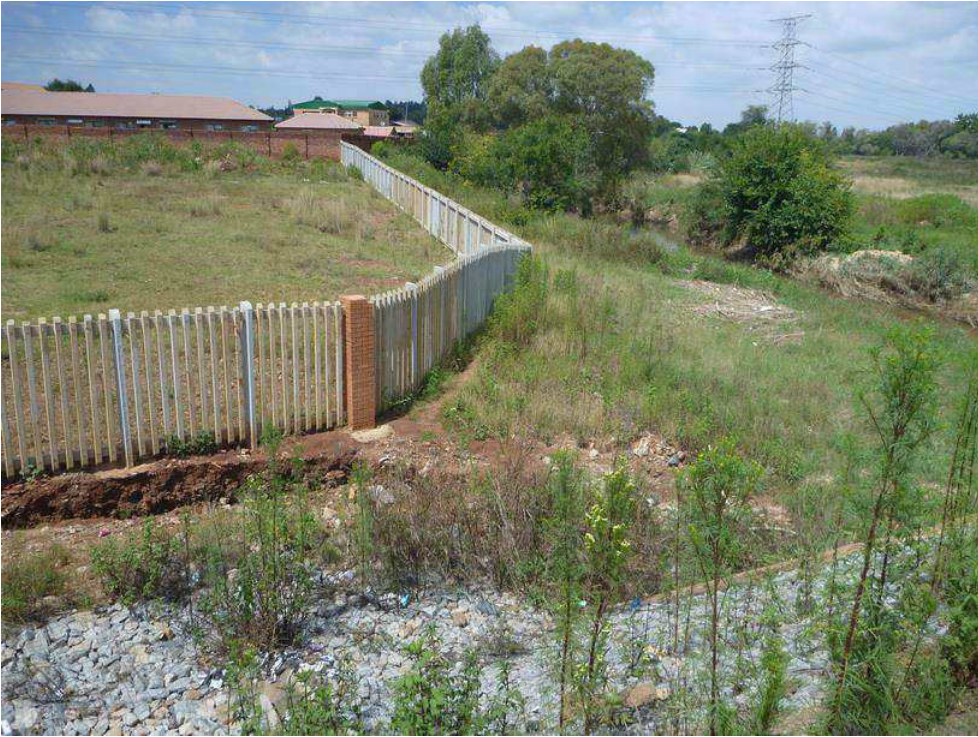
Figure 13 Fence and gabion structures on the banks of the Rietspruit at the R55 river crossing (eastern side)
