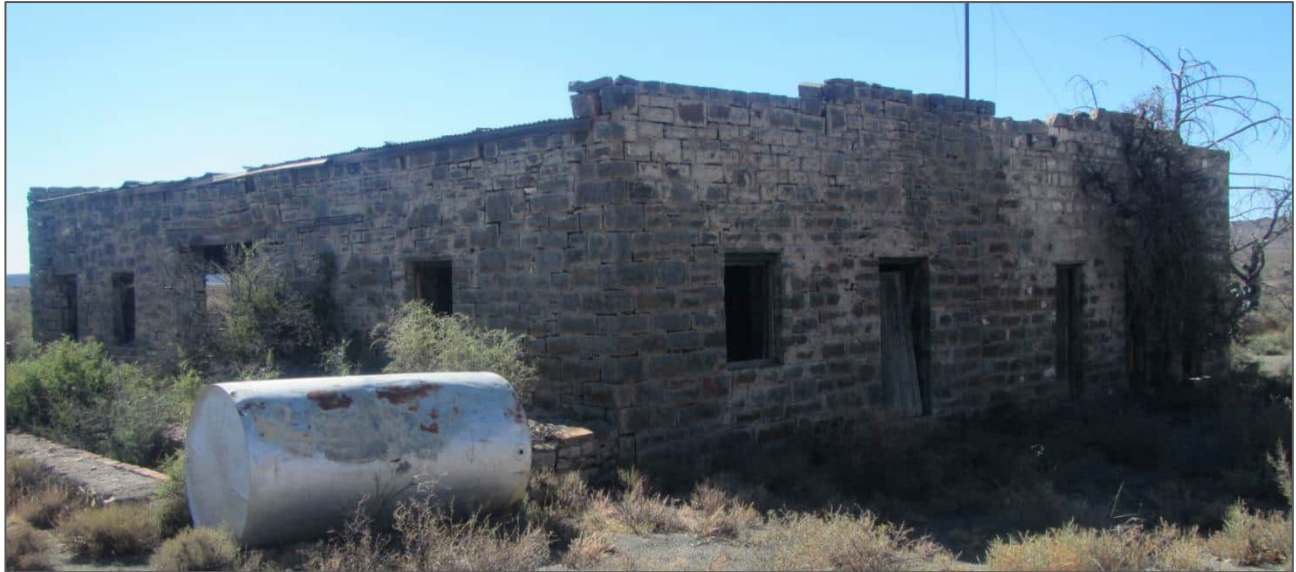
Figure 7-75: A derelict outbuilding alongside the main house at waypoint 1791 in HL04.
