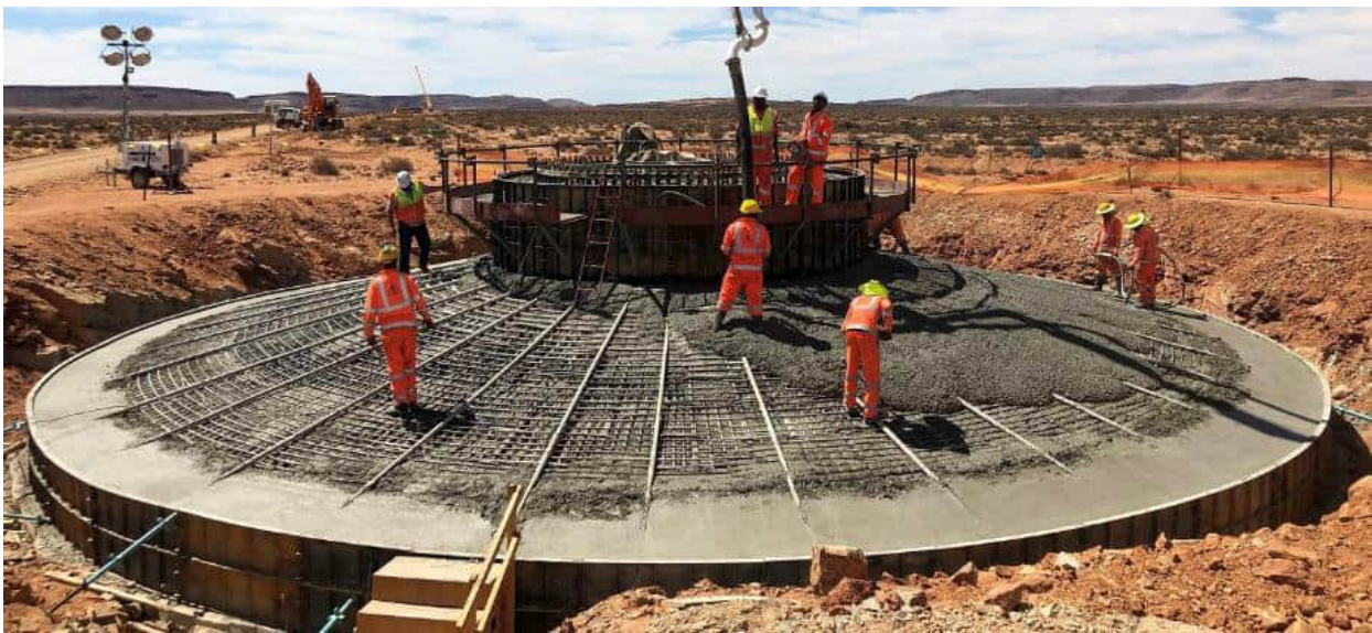
Figure 2-10: Example of a typical turbine foundation under construction
