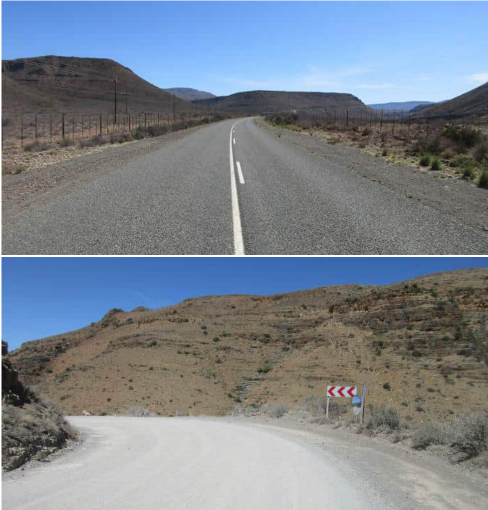
Figure 7-91: Paved and gravel sections of the R381 which will provide the main access to the site via Beaufort West
