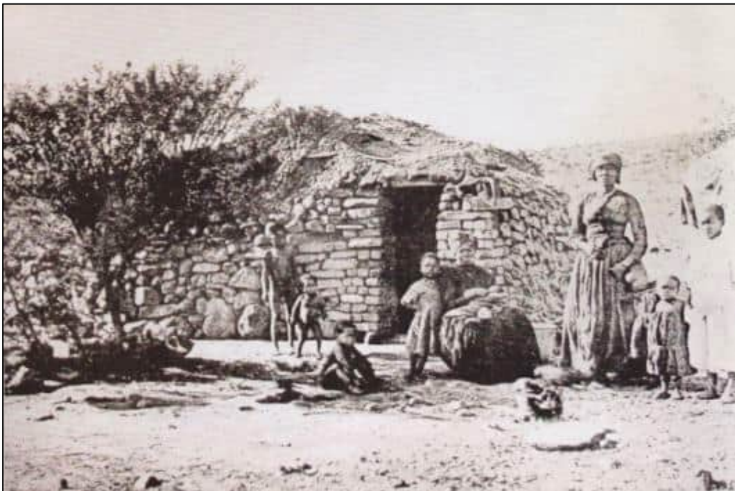
Figure 7-58: A shepherd's hut photographed near Beaufort West in the early 20th century. Note the low, narrow doorway and informal roof structure. Source: Schoeman (2013:48)
