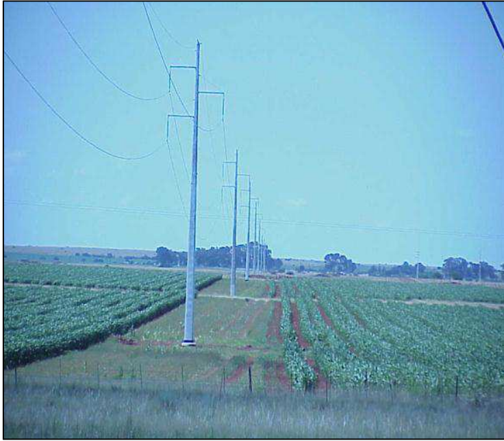
Figure 2: Single Steel Pole Tower Type
