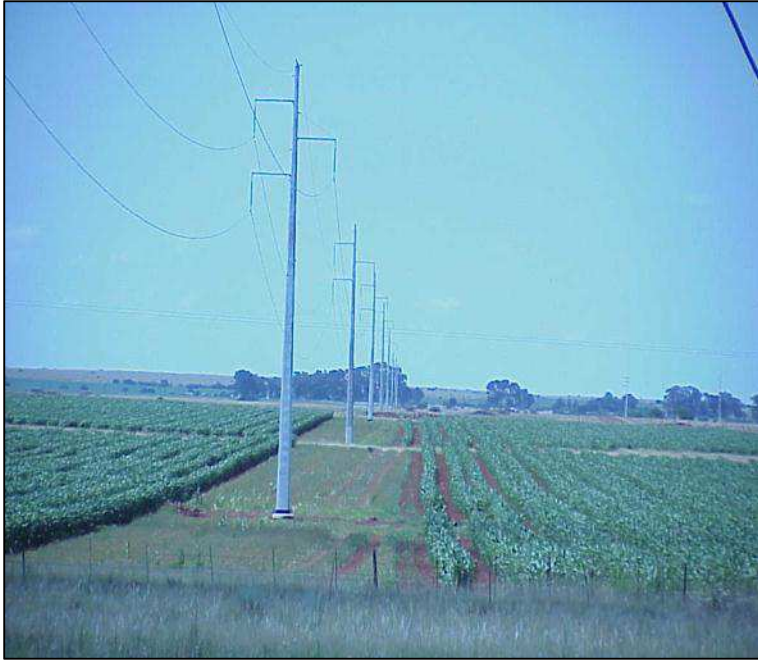
Figure 1: Single Steel Pole Tower Type
