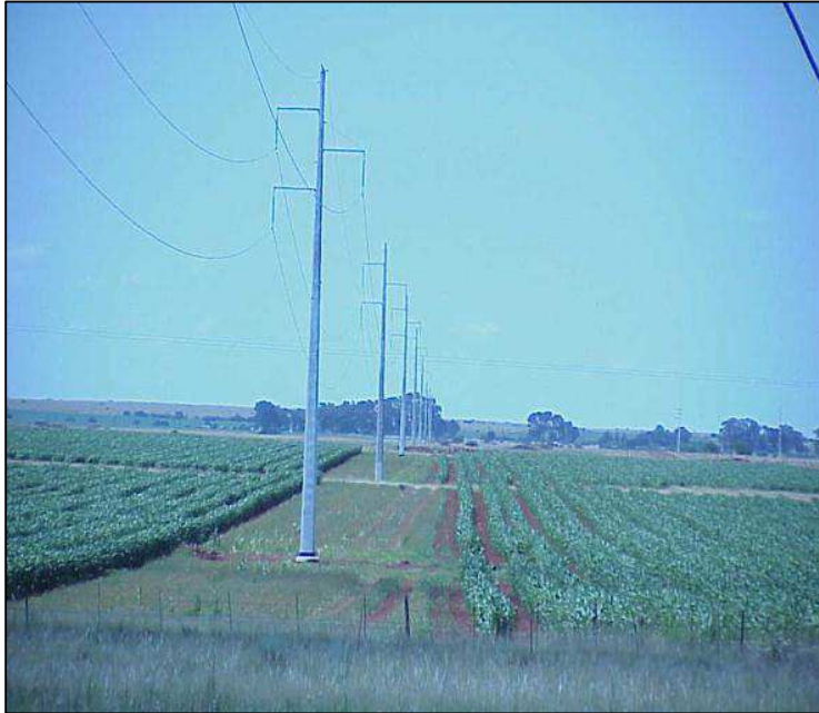
Figure 1: Single Steel Pole Tower Type
