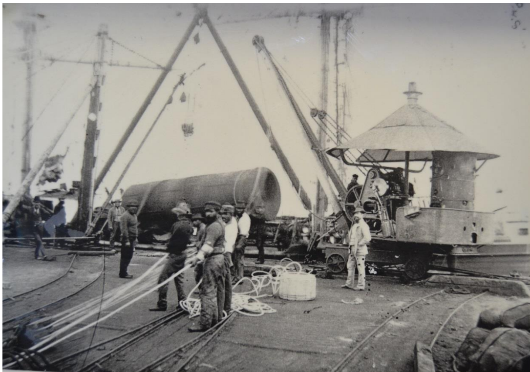
Figure 11: Picture of a mobile steam crane and vertical boiler, taken by H.R Moffatt circa 1880. Courtesy of the Port Nolloth Museum.
