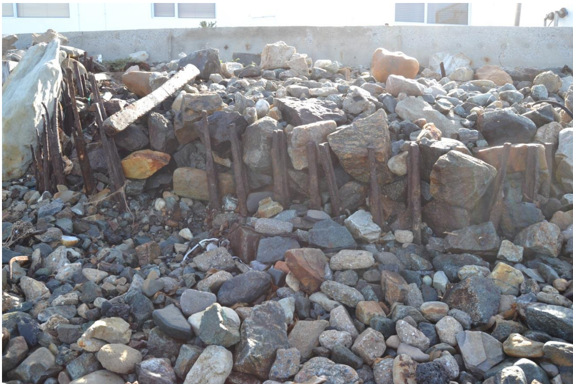
Figure 7: Old railway rails reused to support and stabilise rock.
