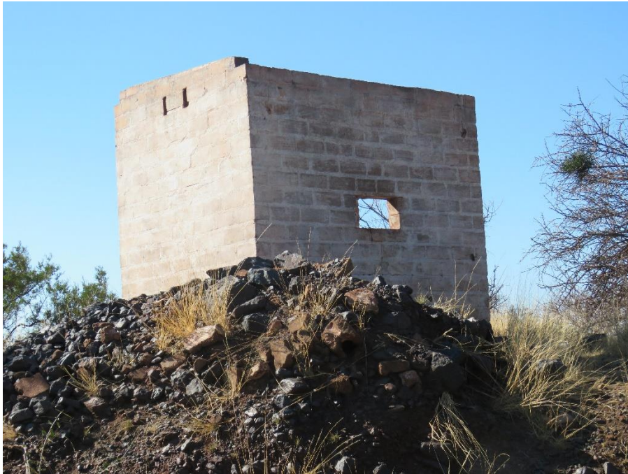
FIGURE 51: ANOTHER ASSOCIATED BUILDING.
