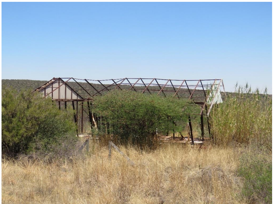
FIGURE 59: STEEL FRAME OF A RAILWAY BUILDING.
