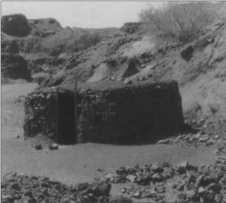
FIGURE 17: HISTORIC PHOTO OF A MINERS BOX, 1920'S (CAIRNCROSS 1997).
