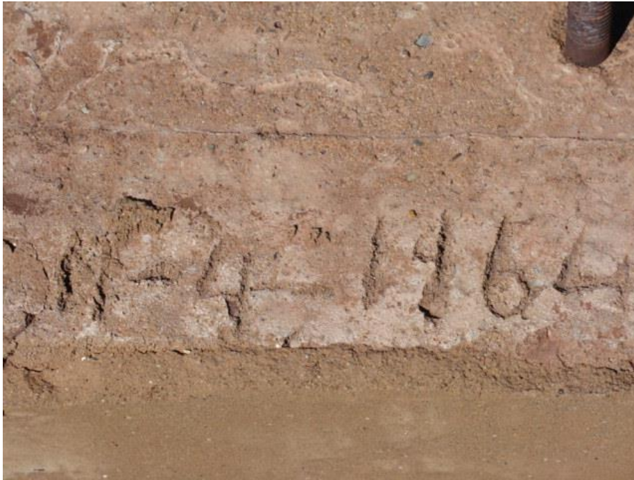
FIGURE 36: (11-4-1964) INDICATED ON THE BUILDING.
