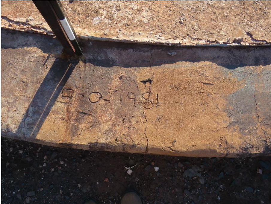
FIGURE 44: DATE INSCRIBED IN THE CONCRETE.
