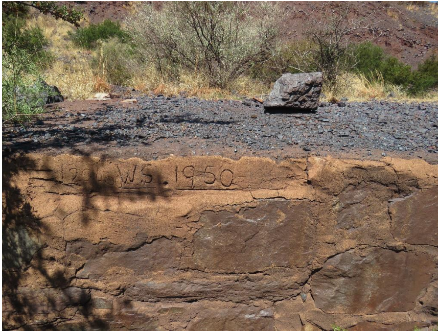
FIGURE 41: DATE (1950) SCRATCHED INTO THE CEMENT OF THE LOADING PLATFORM.
