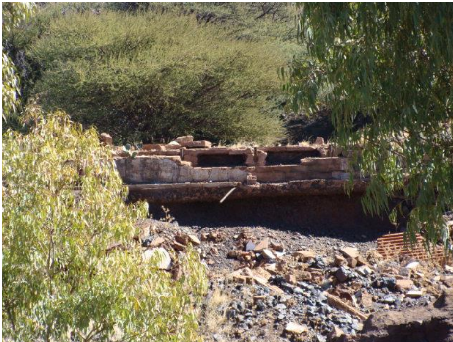
FIGURE 48: REMAINS OF ONE OF THE OTHER BUILDINGS IN THE AREA.
