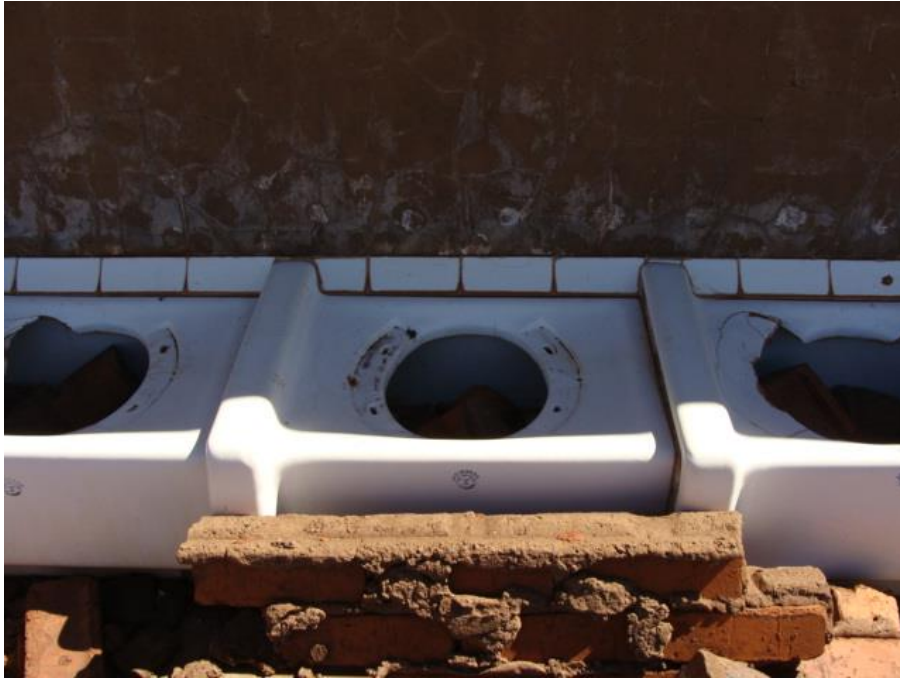
FIGURE 47: PART OF THE ROW OF TOILETS INSIDE OF THE BUILDING.
