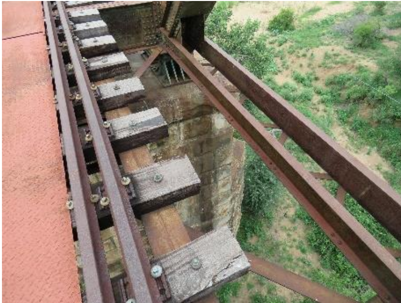
FIGURE 28: DETAILED VIEW OF ONE OF THE PILLARS OF THE BRIDGE.
