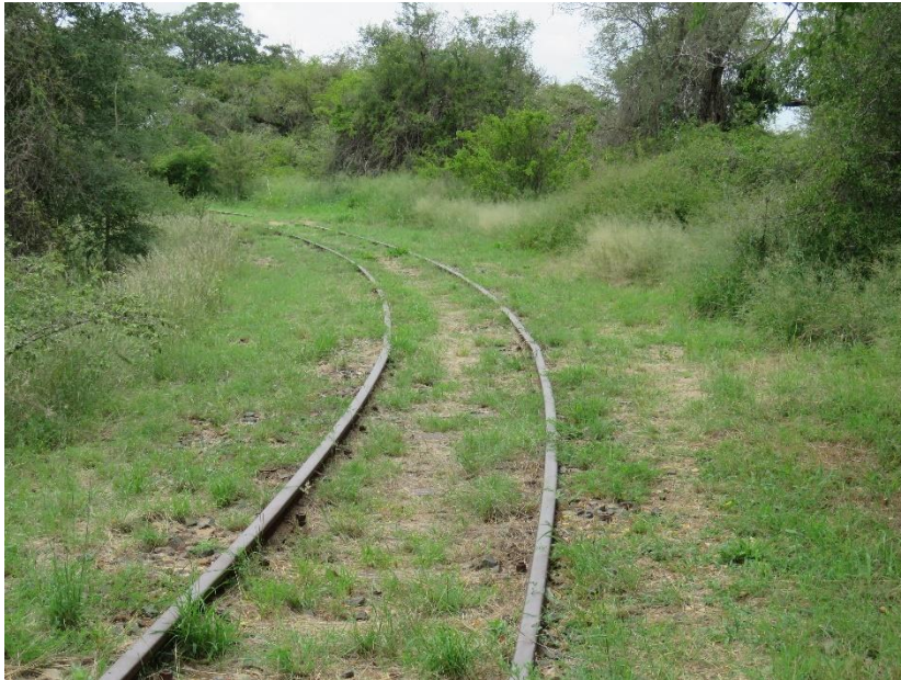
FIGURE 19: EXISTING RAILWAY TRACK BETWEEN THE RESTAURANT AND THE BRIDGE.
