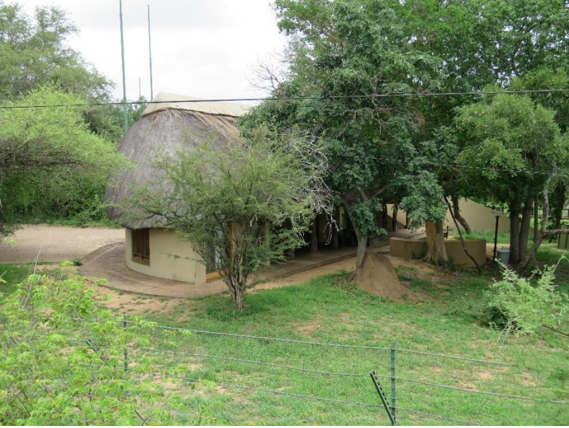
FIGURE 17: WATERKANT GUEST HOUSE.
