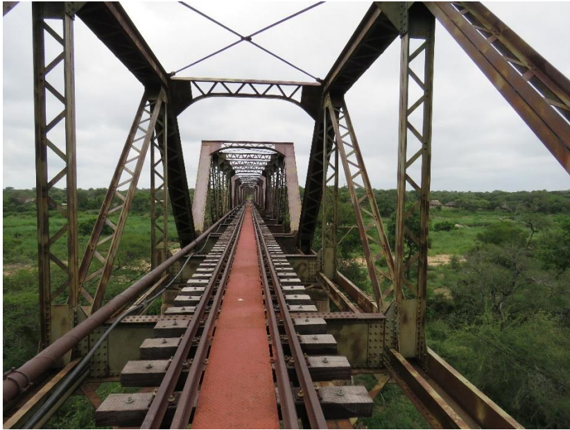
FIGURE 26: DETAILED VIEW OF THE BRIDGE.
