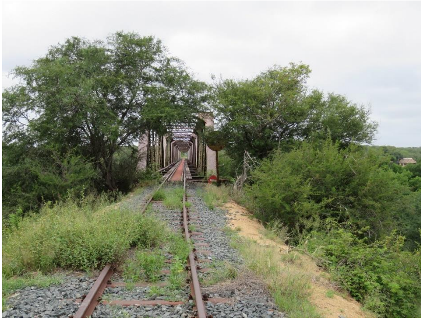
FIGURE 24: NORTHERN VIEW OF THE RAILWAY BRIDGE.
