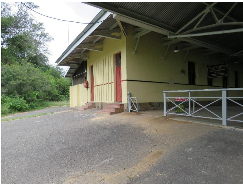
FIGURE 14: EASTERN ENTRANCE TO SELATI RESTAURANT. THE ELECTRICITY TRANSFORMER IS JUST TO THE EAST THEREOF.
