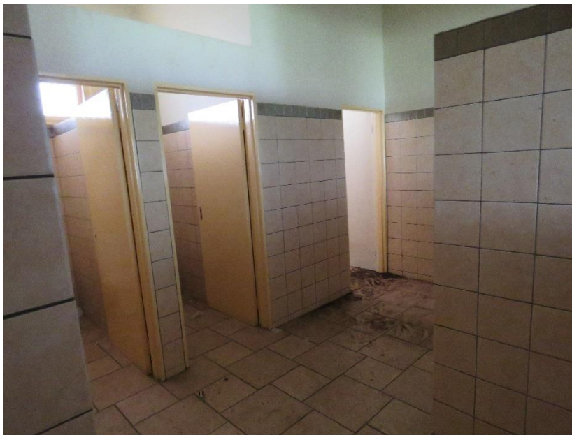
FIGURE 16: TOILET FACILITIES IN RESTAURANT.
