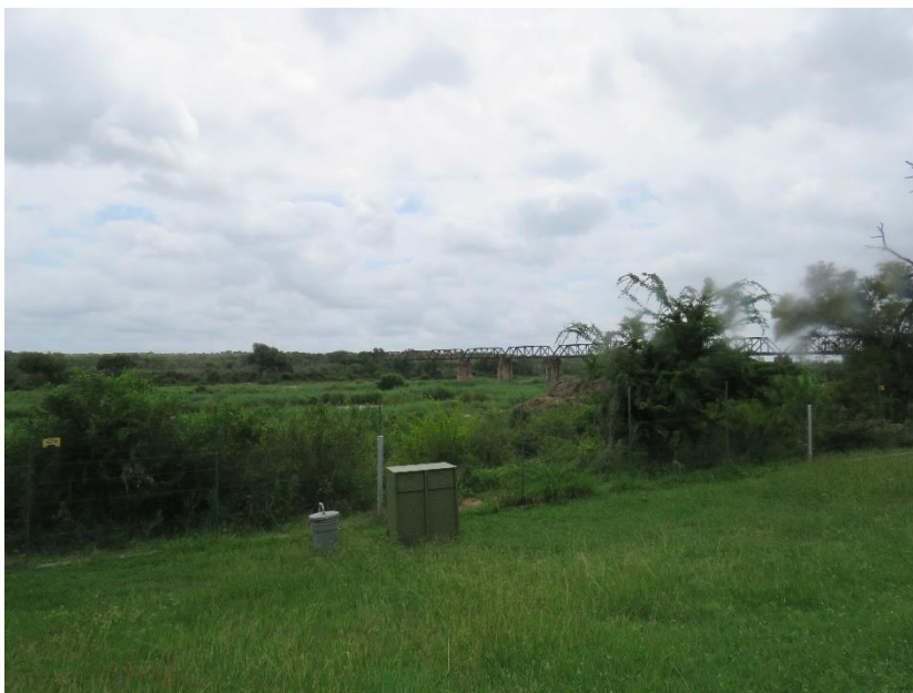
FIGURE 25: VIEW OF THE RAILWAY BRIDGE TAKEN FROM SKUKUZA (SOUTH-WEST).
