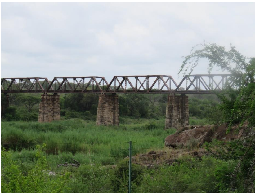
FIGURE 27: NOTE THE SANDSTONE PILLARS OF THE BRIDGE.
