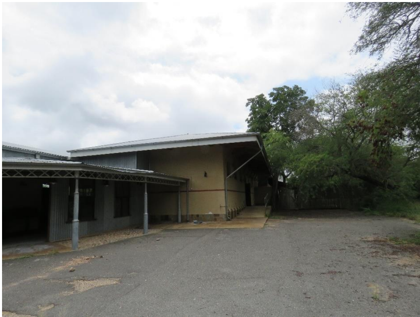
FIGURE 10: ENTRANCE TO THE SELATI RESTAURANT, BUILT DURING THE 1980'S.
