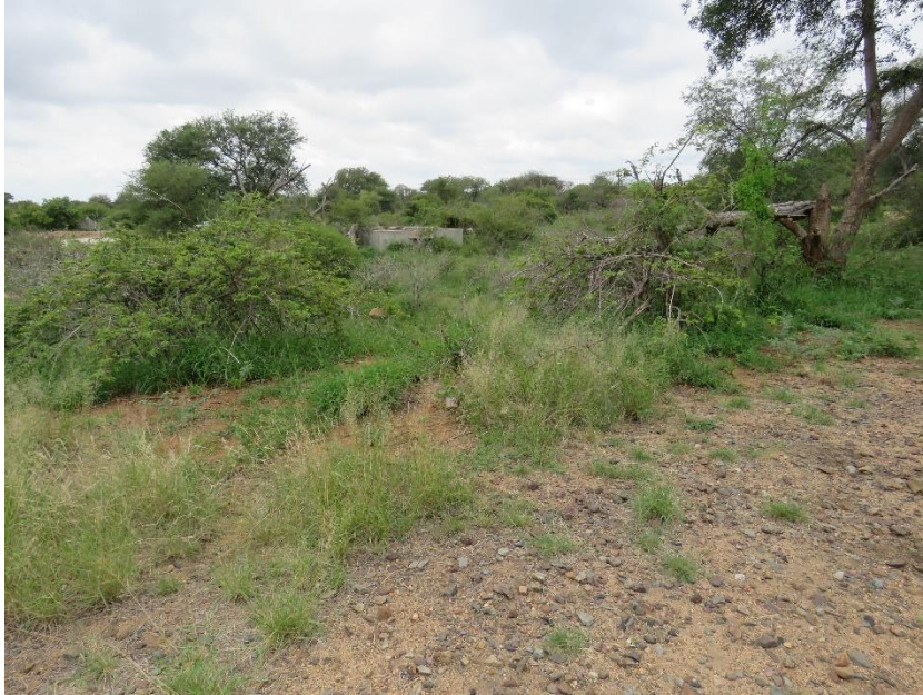
FIGURE 21: ACCESS TO THE BRIDGE ON THE SOUTHERN SIDE OF THE RIVER. NOTE THE CONCRETE STRUCTURE WHICH FORMS PART OF THE WATER PUMPING SYSTEM.
