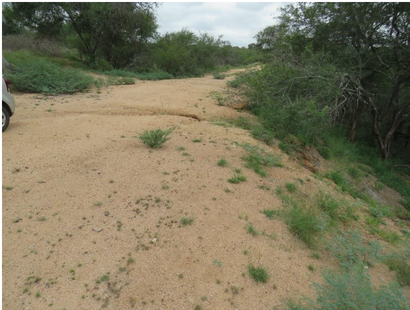
FIGURE 22: ACCESS TO THE BRIDGE ON THE NORTHERN SIDE OF THE RIVER.
