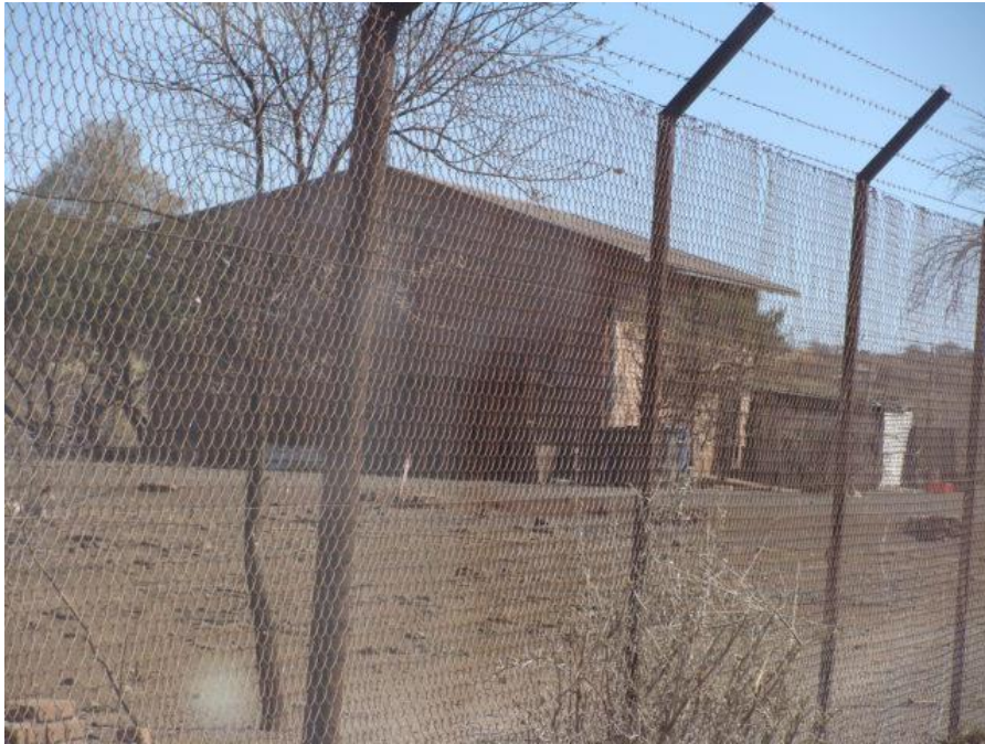
FIGURE 63: ONE OF THE BUILDINGS INSIDE OF A FENCED IN CATTLE CAMP.
