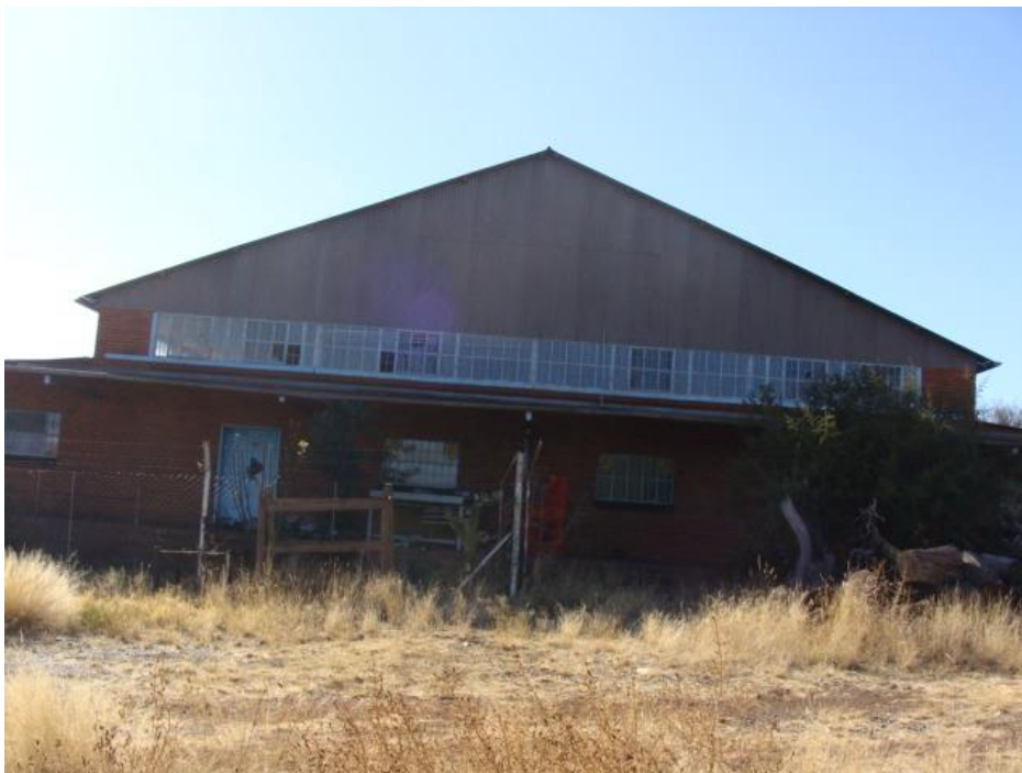
FIGURE 32: OLD RECREATION HALL CLOSE TO THE HOSTEL AREA.
