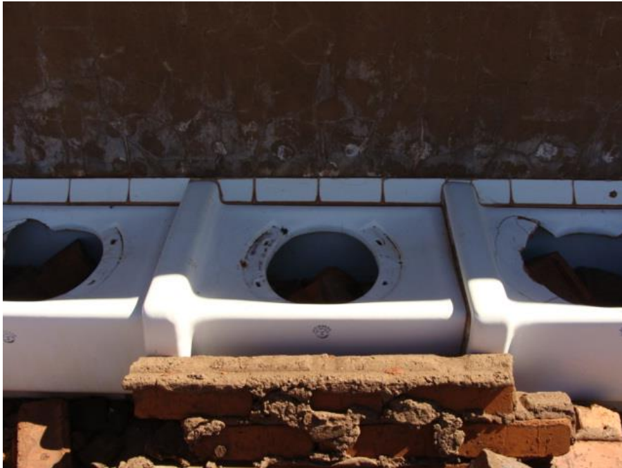
FIGURE 56: PART OF THE ROW OF TOILETS INSIDE OF THE BUILDING.
