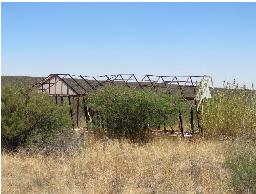
FIGURE 68: STEEL FRAME OF A RAILWAY BUILDING.
