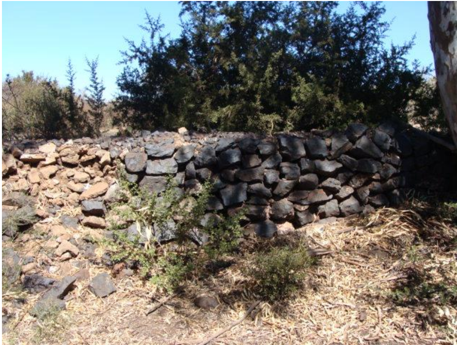
FIGURE 58: STONE WALL IN THE AREA.
