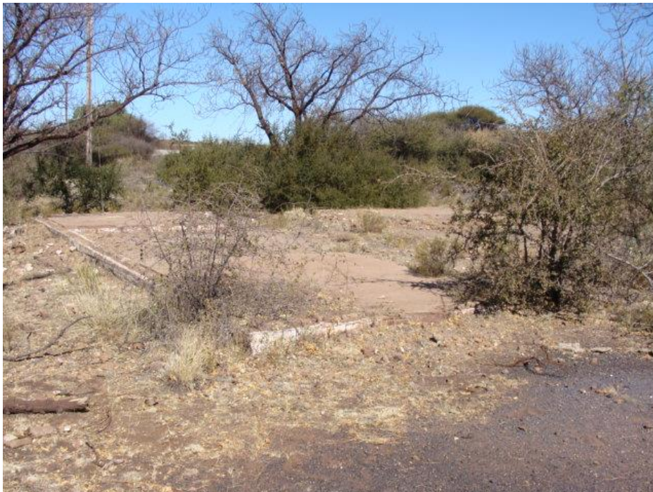
Figure 43: Foundation of a building more than 60 years old.
