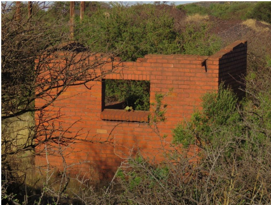
FIGURE 46: SECOND BUILDING ASSOCIATED WITH THE FIRST.
