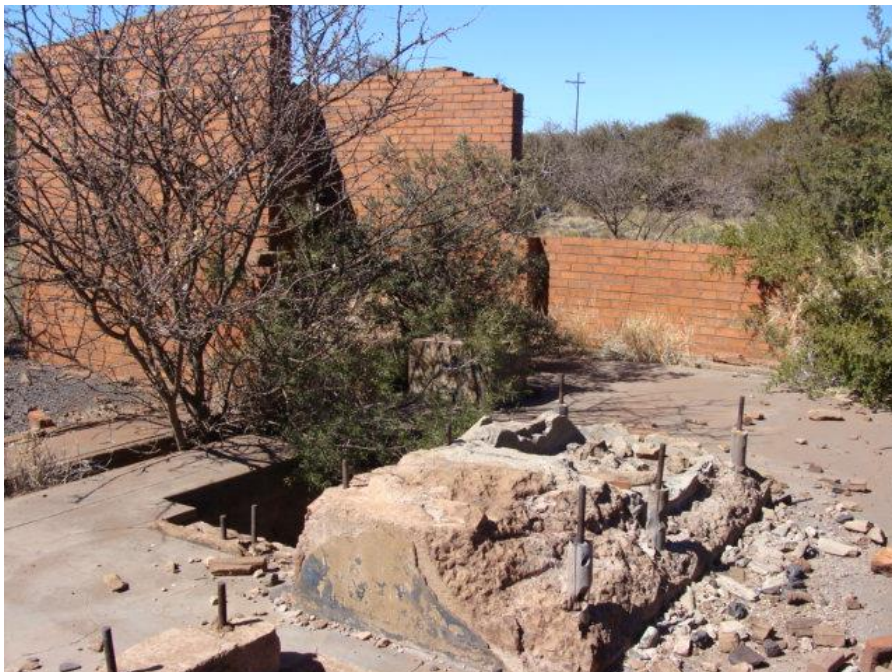
FIGURE 44: REMAINS OF AN INDUSTRIAL BUILDING IN THE MINING AREA.
