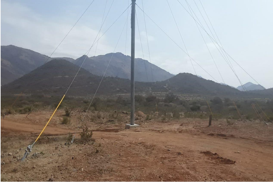
Figure 12: View proposed pylon site 74 next to construction of another powerline.
