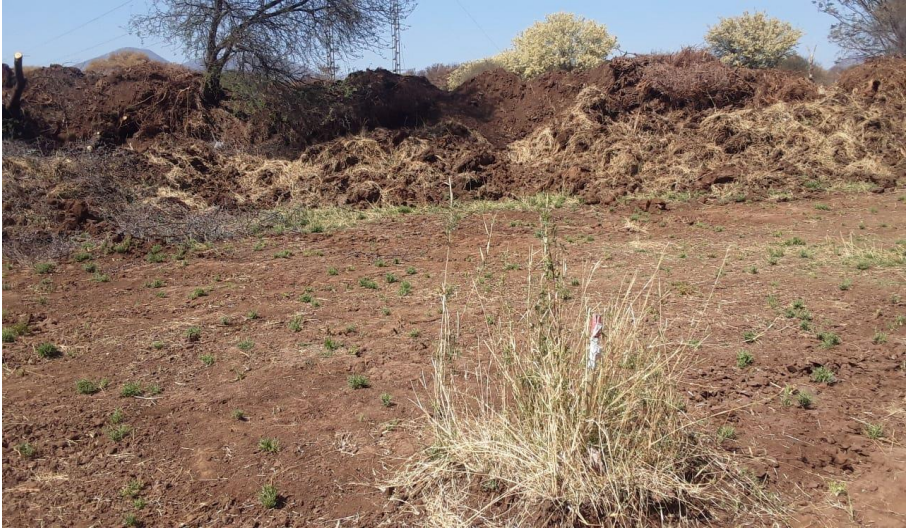
Figure 10: View of vegetation clearing at proposed pylon site 20.
