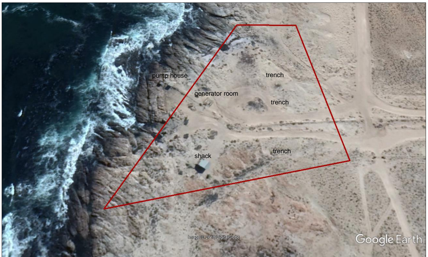
Figure 4. Google satellite image of the subject property including existing infrastructure. Note the extremely degraded context of the site
