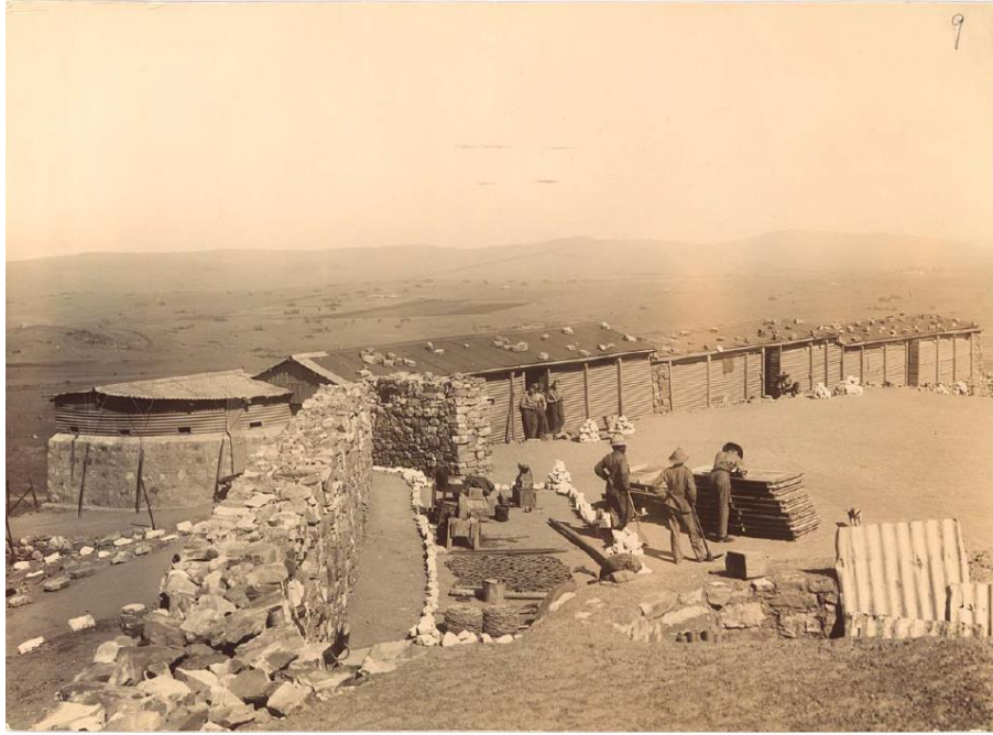
Figure 78: Photograph of the East Fort during the War. Note the corrugated iron buildings. Also note the loopholes in the structure to the left (British National Archives, WO/108/342, p. 9).
