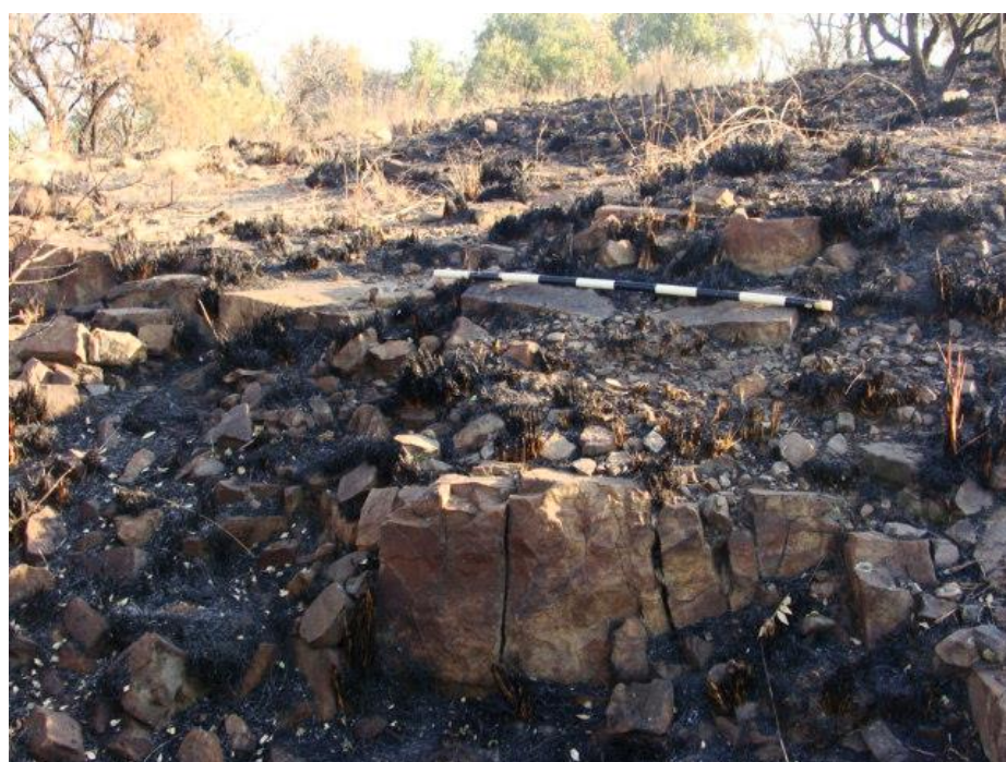
Figure 8: Corner junction between wall on the western and one on the southern side.
