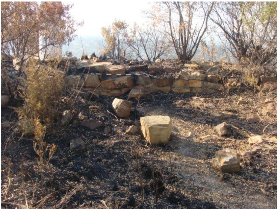
Figure 14: Remains of a circular wall where a blockhouse may have been placed.
