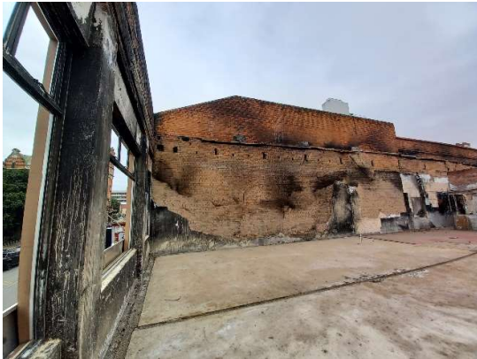
Figure 10: Front facade and adjacent parapet wall
