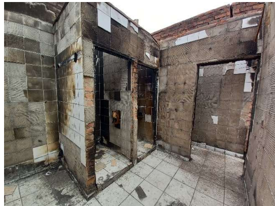
Figure 13: Internal view of ablutions
