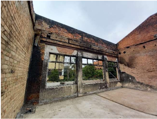
Figure 8: Internal view of front facade
