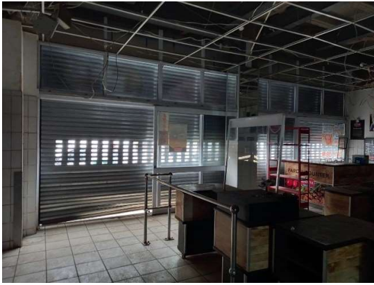
Figure 14: Ground Floor Shop
