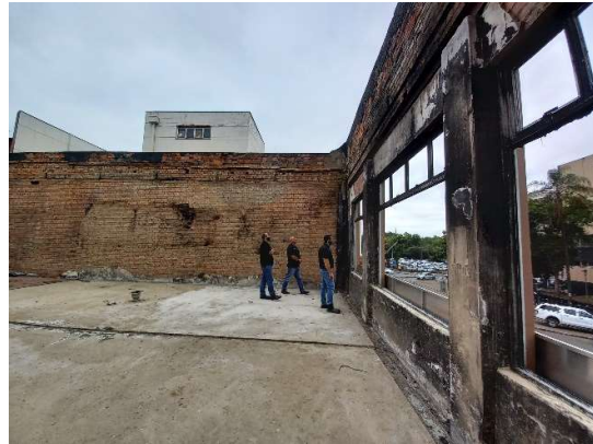
Figure 11: Front facade and adjacent parapet wall
