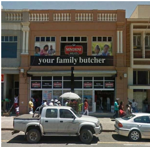
Figure 1: 287 Church Street Before Fire Damage
