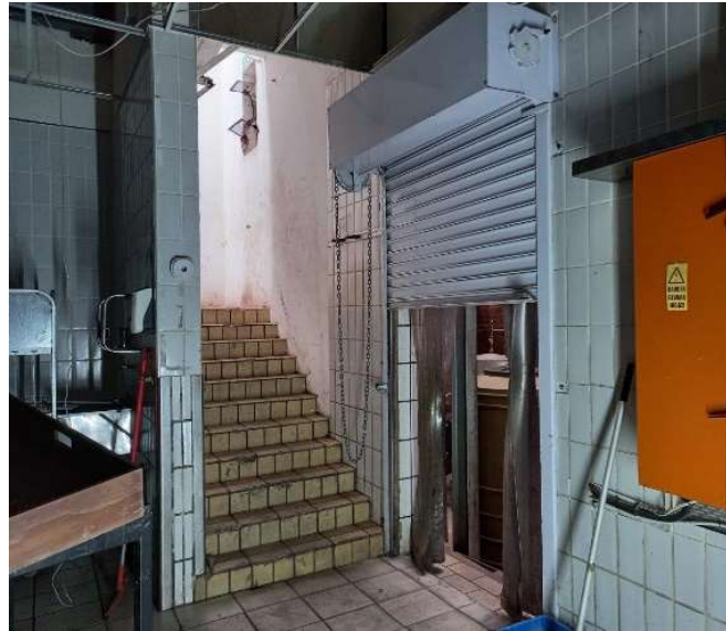
Figure 17: Delivery Entrance from ROW servitude
