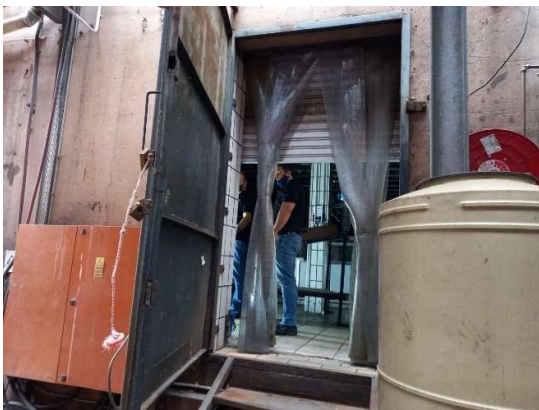
Figure 18: Delivery Entrance from ROW servitude
