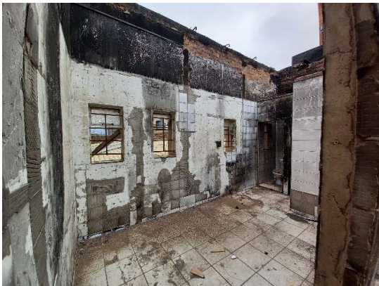
Figure 12: Internal view of ablutions
