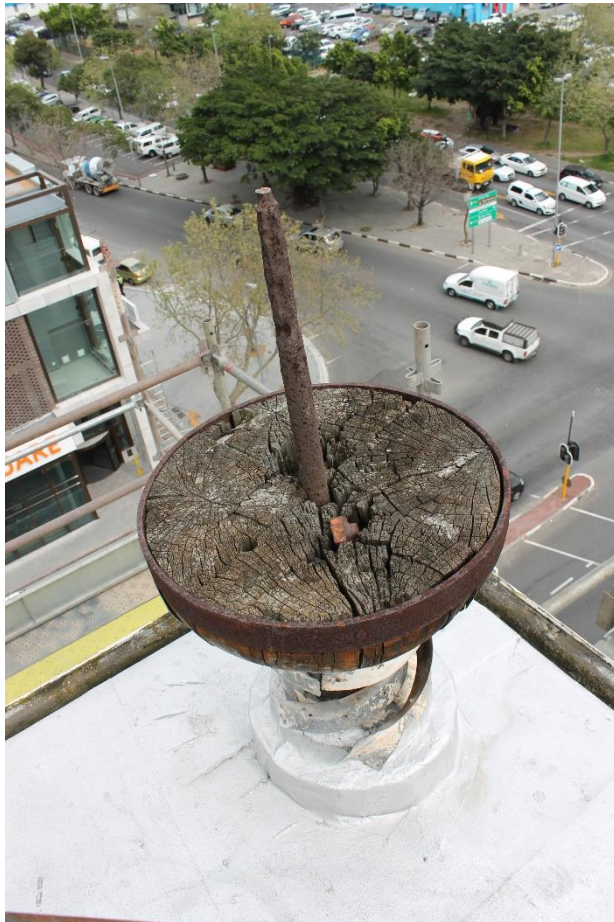
The first urn which has lost the top half and is showing serious rot in the remaining bottom half.
