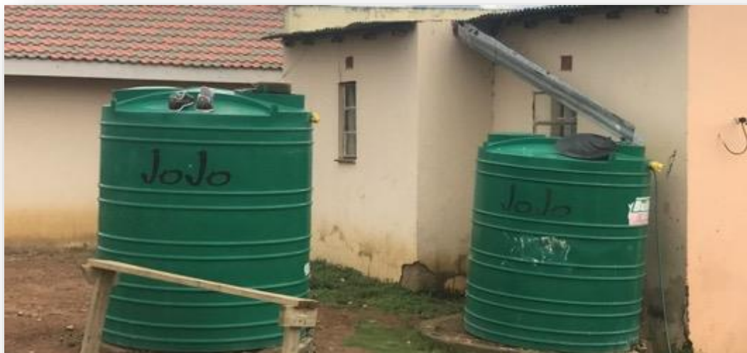
Figure 27: Jojo tanks used to store water
