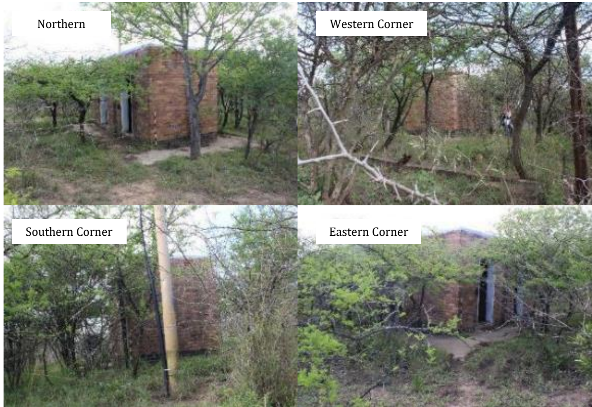
Figure 33: View of the 4 corners of Transnet House-01 structure
