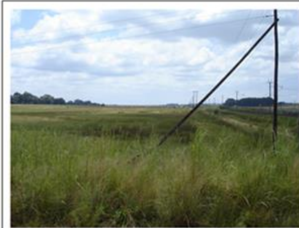
Figure 3: A small seepage area alongside the N4; a typical sight in the area.
