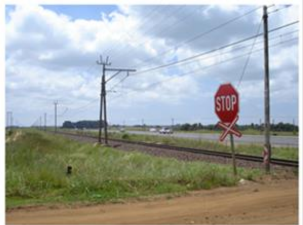
Figure 4: Railway and telecommunication infrastructure.
