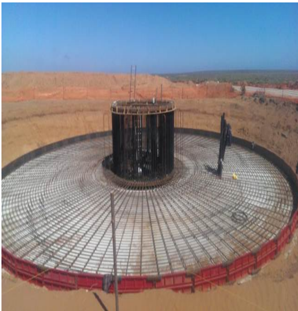
Figure 7.1: Concrete foundation (Eskom Sere Wind Facility)
