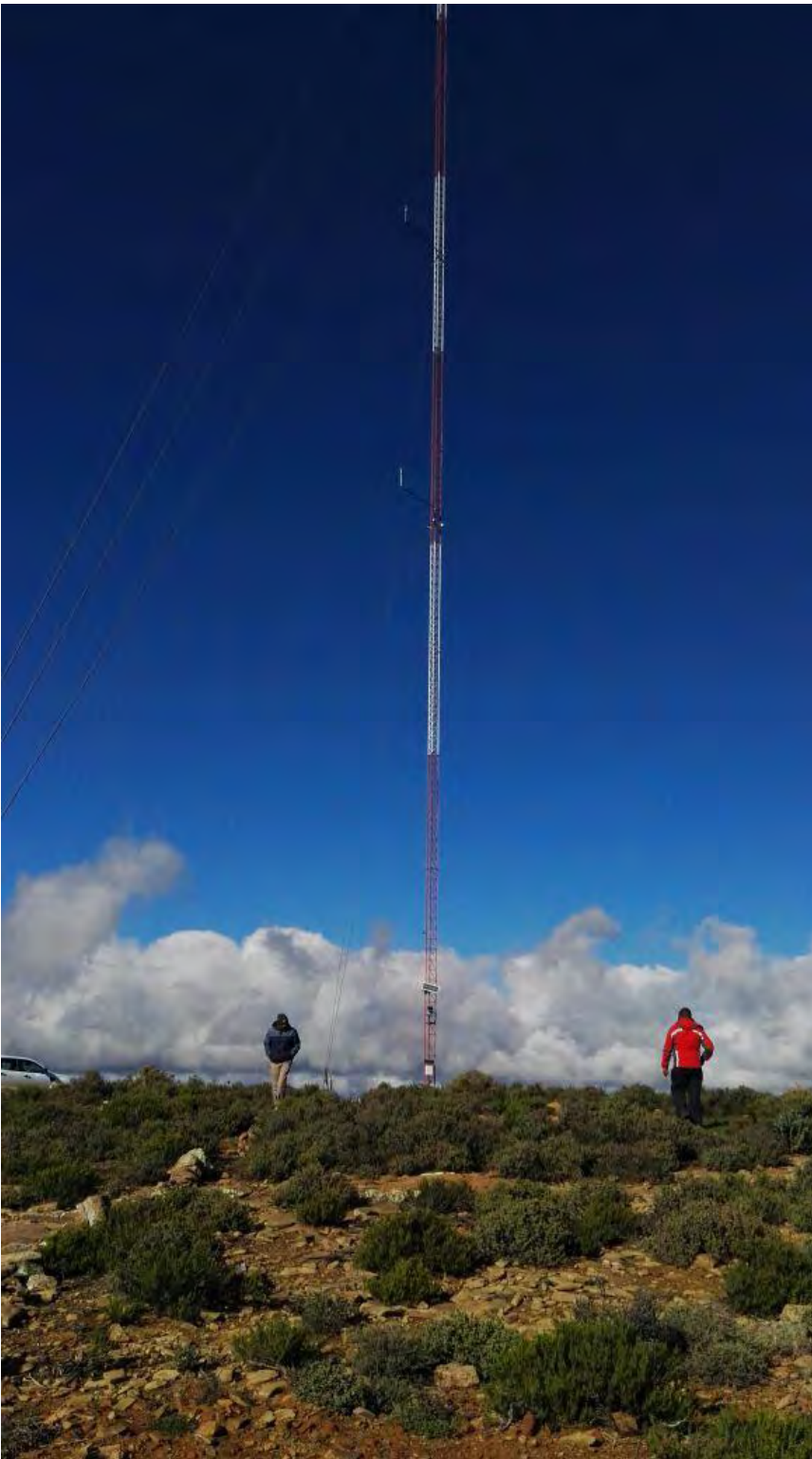
Plate 2-1: An example of a meteorological mast.
