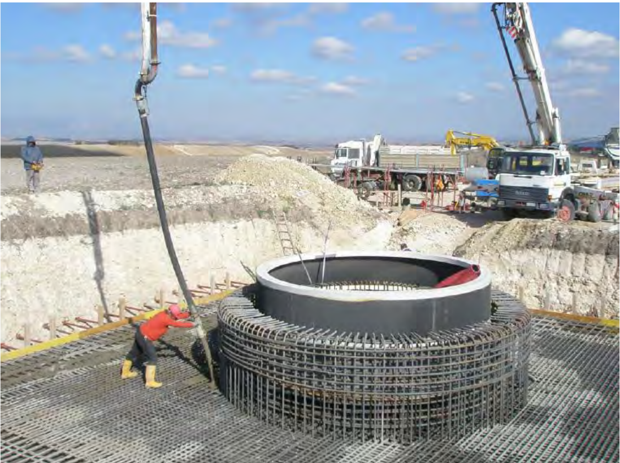
Plate 2-2: Concrete pouring of a turbine foundation – note the tower base collar in the foreground.
