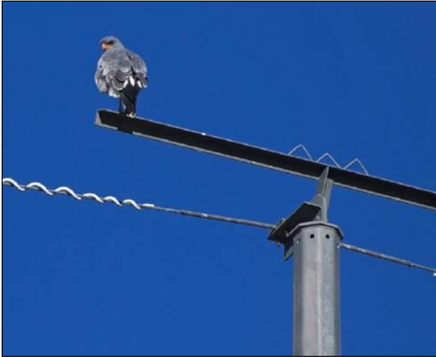
Photograph 6. A Pale Chanting Goshawk ( Melierax canorus ) perched safely on a 'Bird Perch' (Photo: EWT-WEP)
