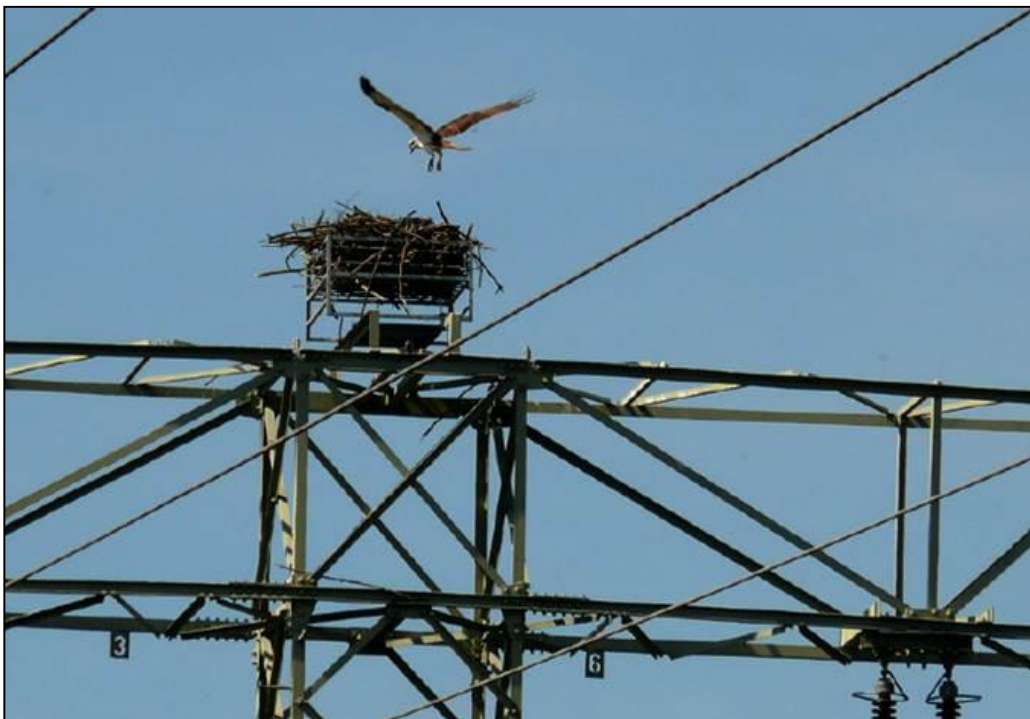
Photograph 7. Nesting Osprey on artificial platform in medium voltage transmission line (Photo; Bureau Waardenburg)
