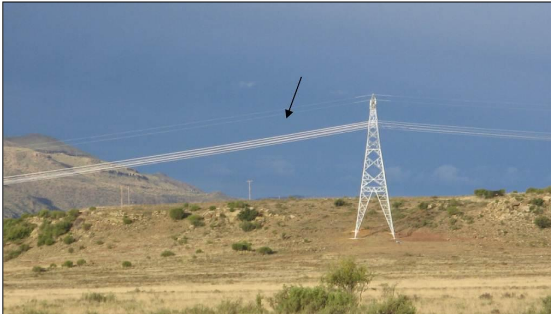
Photograph 9. A 400 kV line, with all conductor wires in the same horizontal plane (Photo: EWT-WEP)
