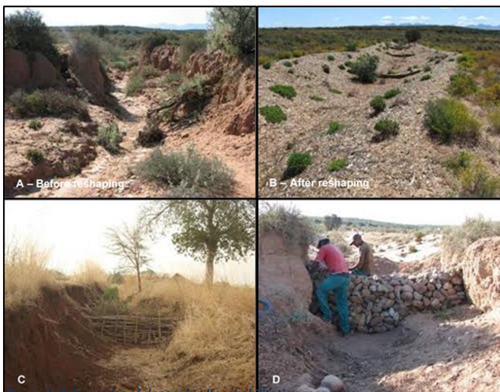
Figure 6-2: Examples of donga / gully rehabilitation measures
