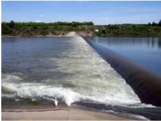
Figure 7 | Example of a weir.
