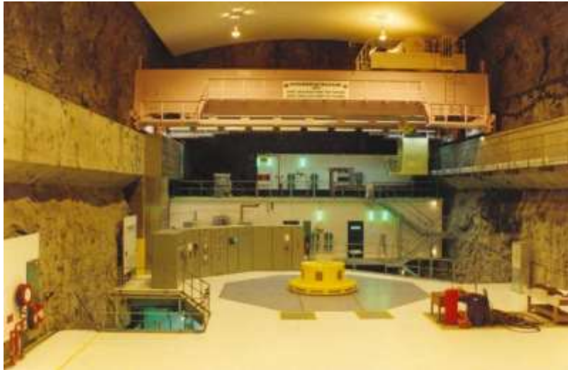
Figure 11 | Example of an Underground powerhouse.
