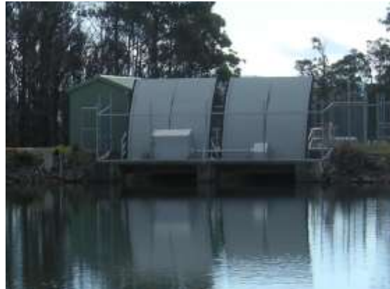
Figure 8 | Example of an intake structure.
