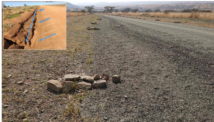
Figure 6-3 Example of road margin erosion prevention
