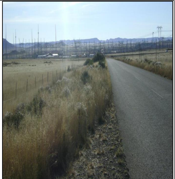
The Hydra Substation in the west of the study area.
