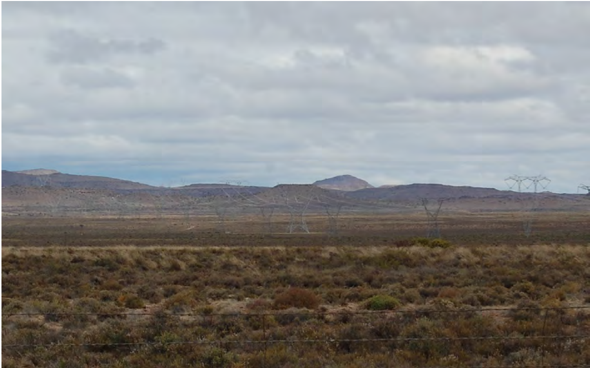
Figure 1-24 High voltage transmission lines with lattice towers against a mottled landscape similar to that of the Sutherland region (photo taken by author).
