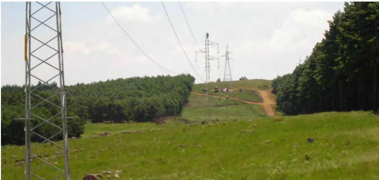
Figure 1-22 An example of lattice towers used for 132 kV power lines. (Source: https://optipower.co.za/mizpah-msingqa/ )
