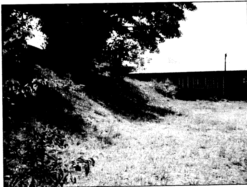
I&AP RECENT PHOTOGRAPH (NOV 2010) SHOWING SECTION OF CUT SLOPE FROM DIFFERENT ANGLE. DEPTH OF CUT SLOPE VARIES BETWEEN APPROXIMATELY ONE AND TWO METRES
