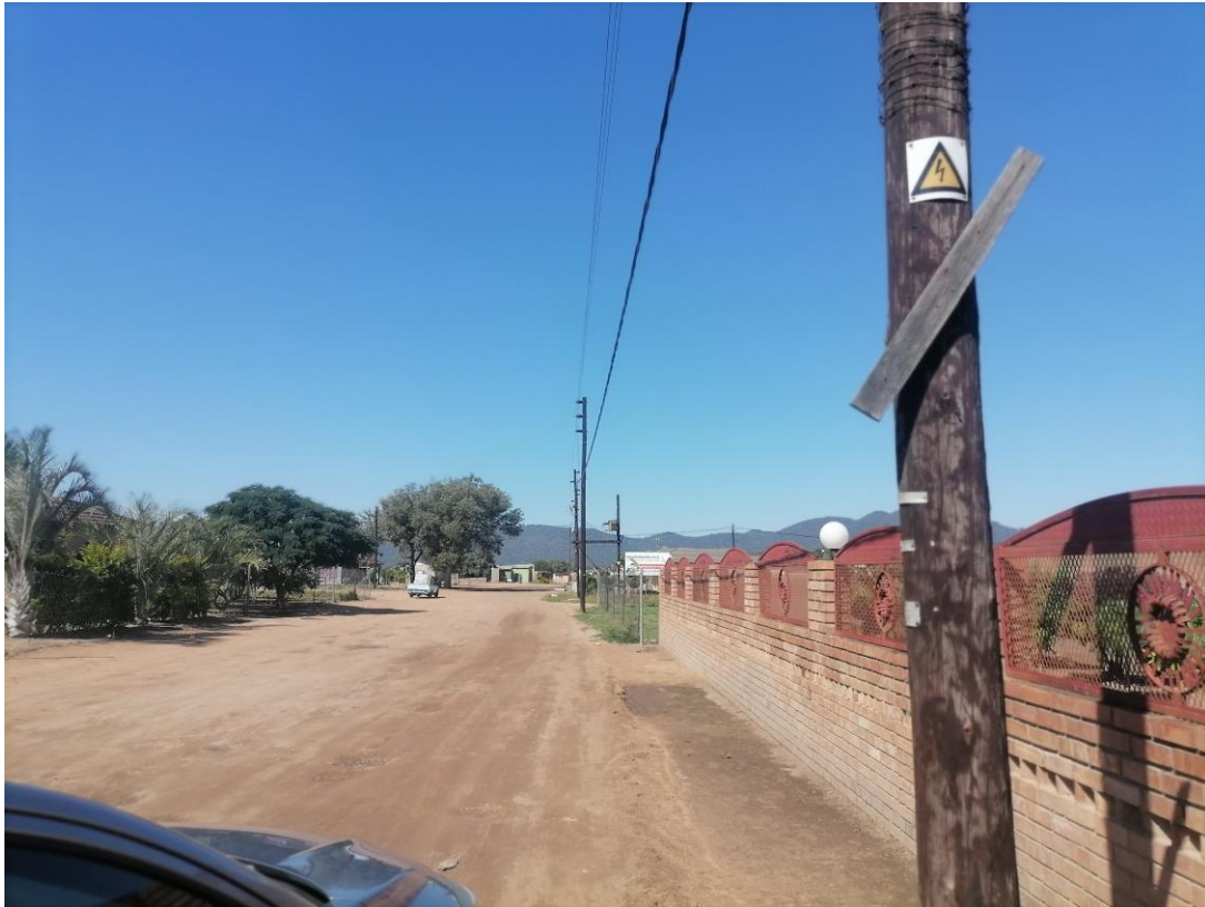
The existing powerlines on site
