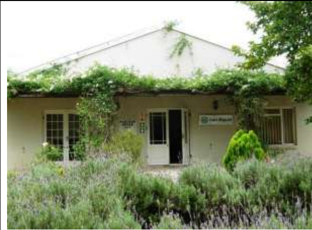
Photo 2.2. Existing River Bend Citrus Farm Offices.
