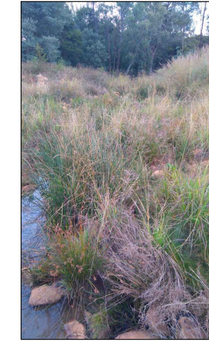
PHOTO 1 TYPICAL BOULDER CHANNEL +/- 1.5 YEARS AFTER CONSTRUCTION COMPLETED N.T.S.
