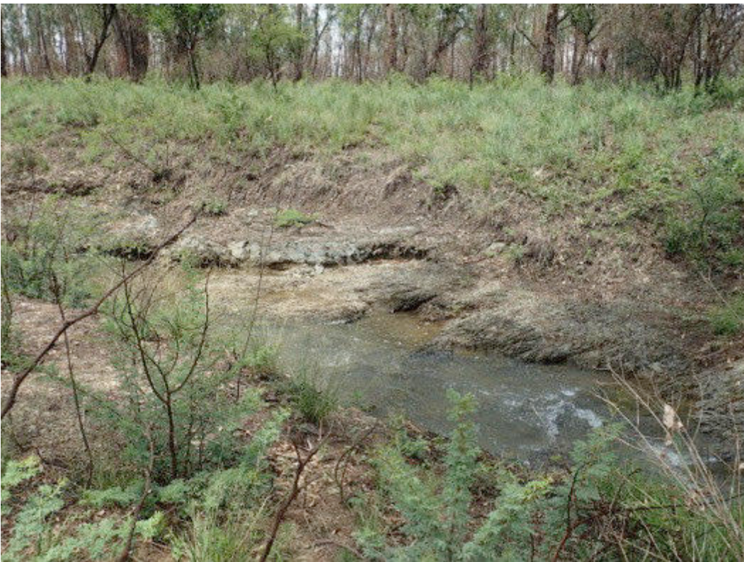
Figure 29 Eroded channel along the watercourse
