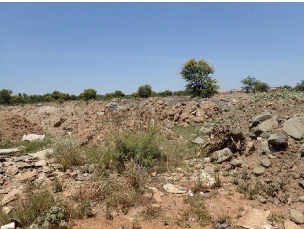
Figure 17 Dumping of rubble on the site
