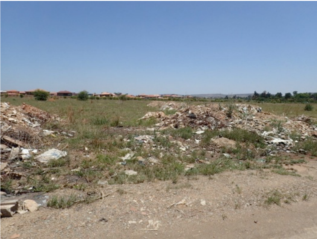
Figure 16 Dumping of rubble on the site
