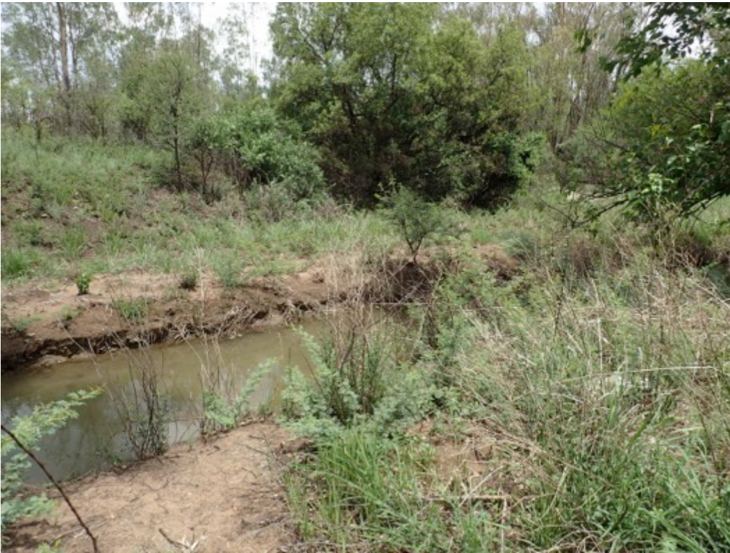
Figure 28 Eroded channel along the watercourse
