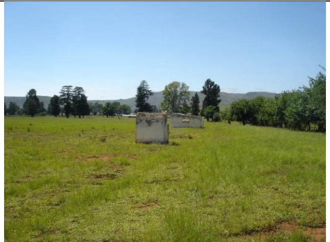
Figure 8. Looking south east showing the remains of the sports ablution facilities.
