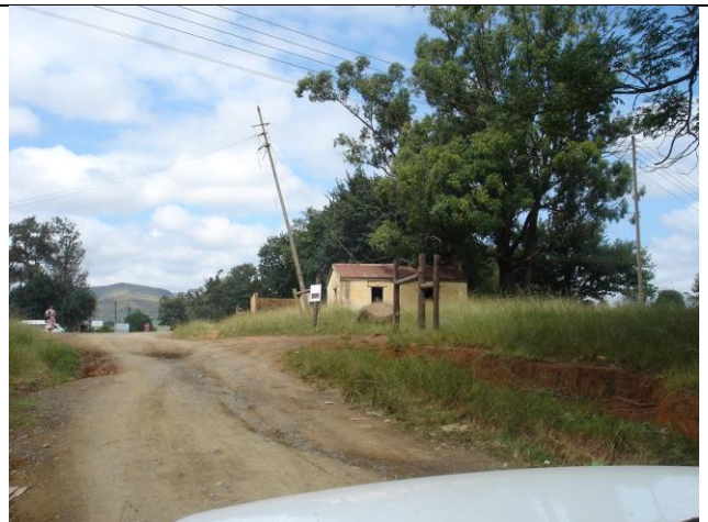
Figure 10. Image showing the existing access road.
