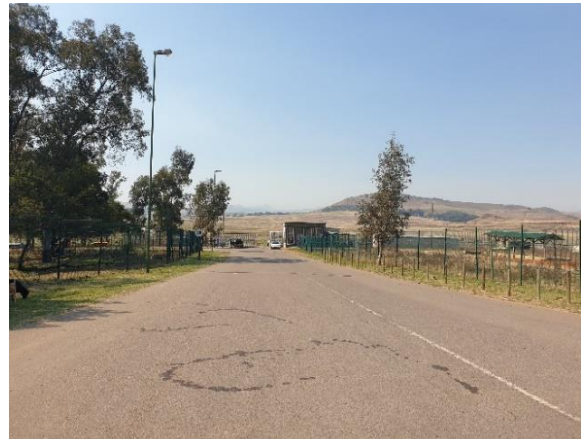
Figure 8: North-east view to the existing access roads to the industrial complex
