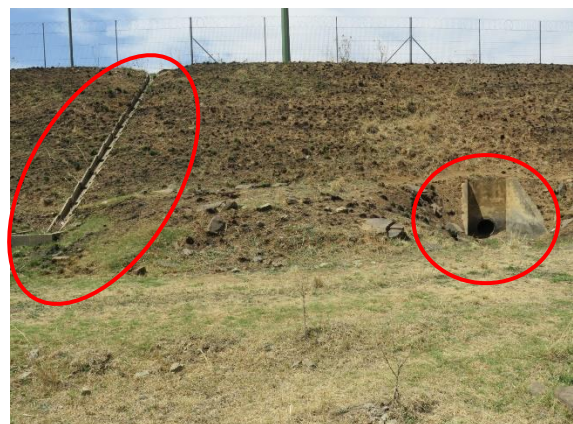
Figure 12: Formalised stormwater management infrastructure on the platform embankment in Figure 11
