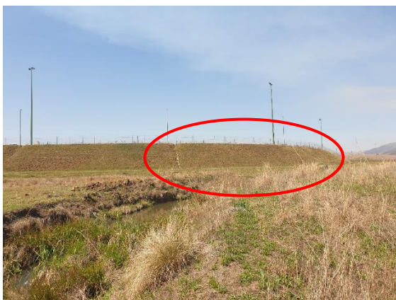
Figure 11: Area proposed for the construction of the culvert across the watercourse
