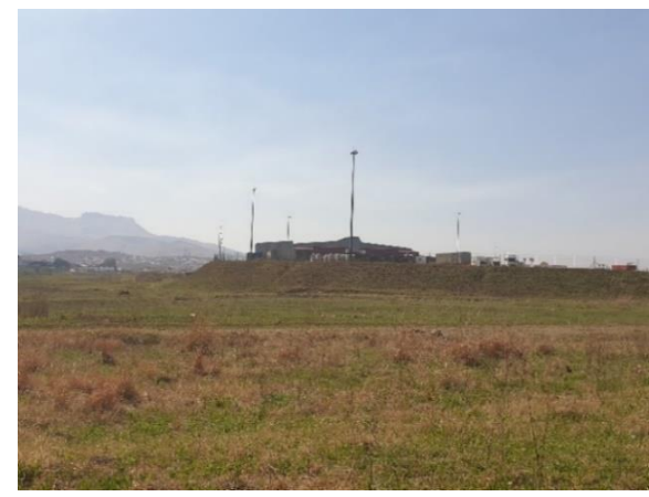
Figure 6: Industrial complex located north-east of the project site
