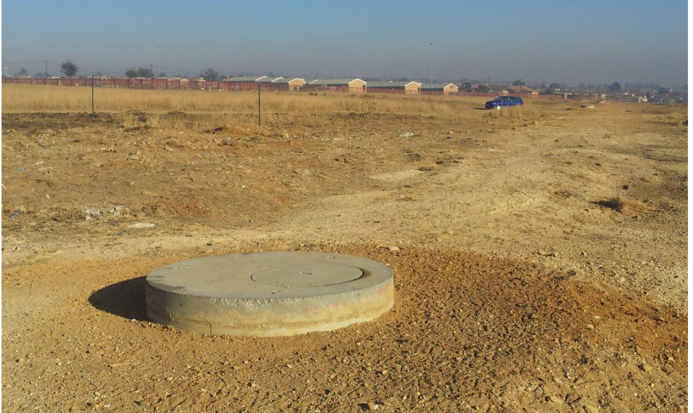
Plate 1: Recently installed sewer line traversing the eastern edge of the site.
