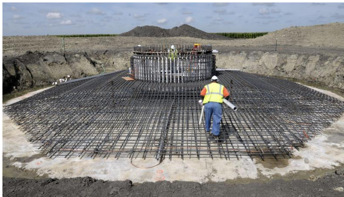
Figure 4.4: Photograph illustrating the construction of the foundation for a wind turbine 9
